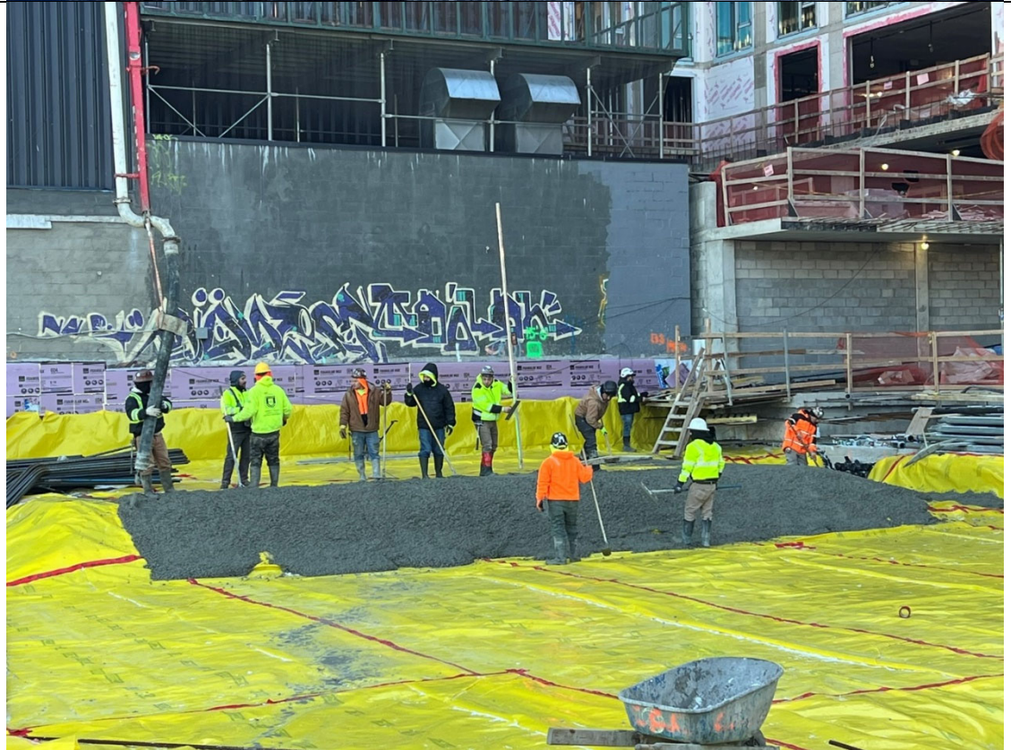
Photo 2- Representative photo of rat slab being poured.
