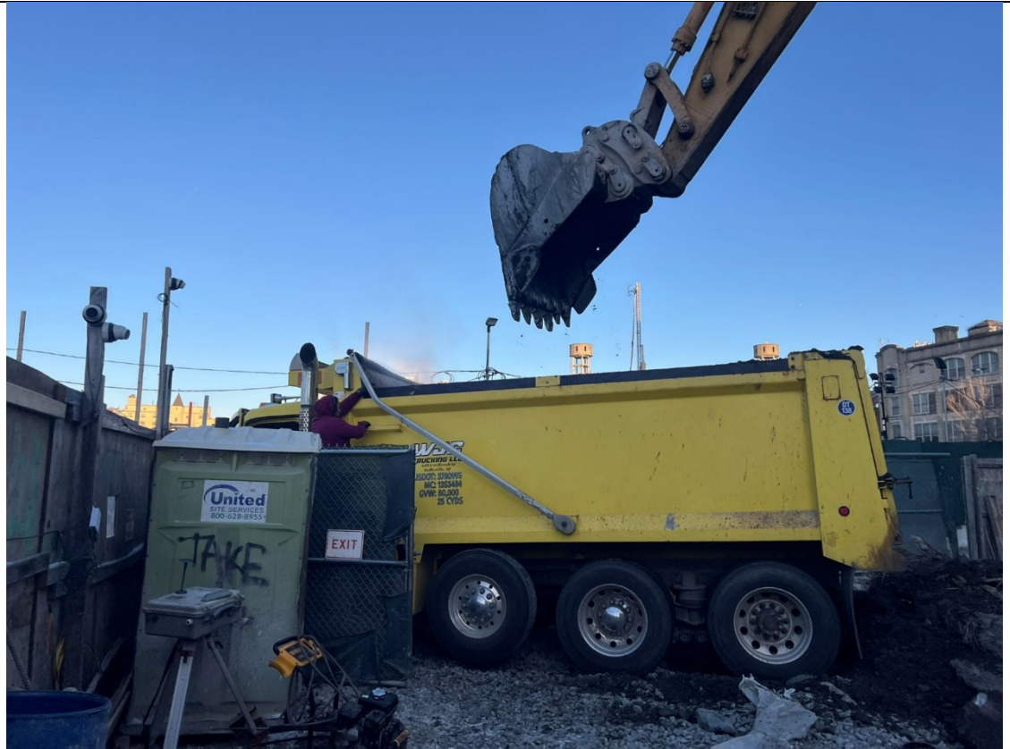
Photo 1- Representative photo of trucking treated material.
