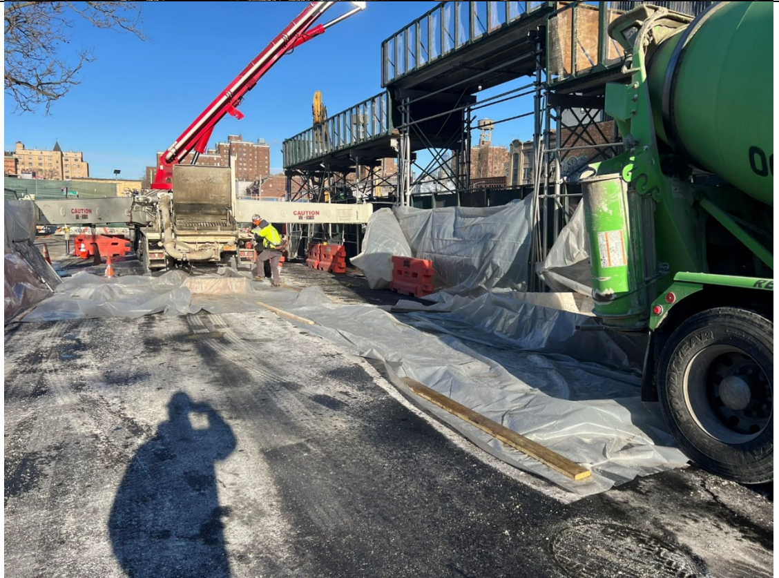
Photo 4- Representative photo of the concrete washout.
