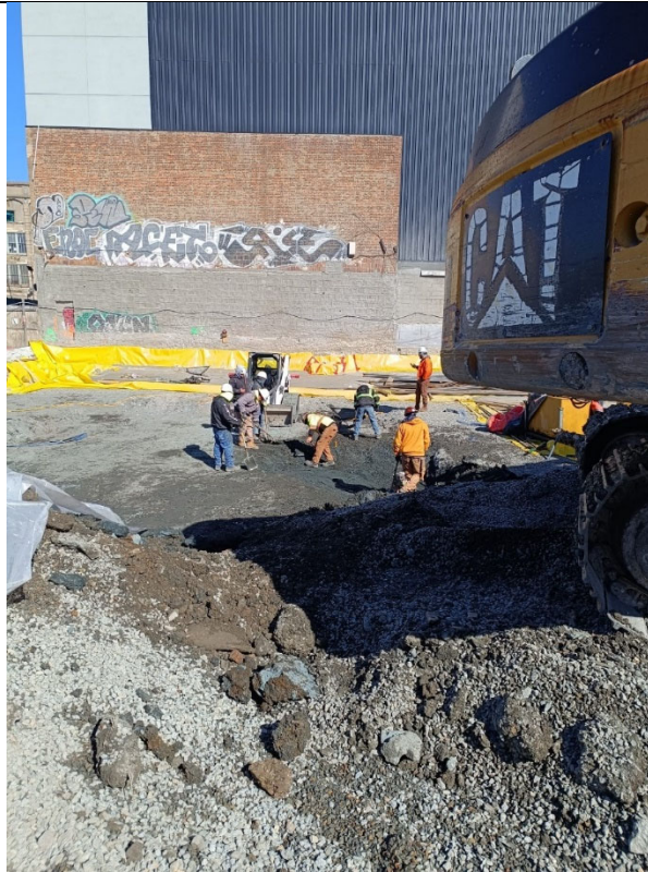
Photo 3- Representative photo of Concrete Course compacting excavated area.
