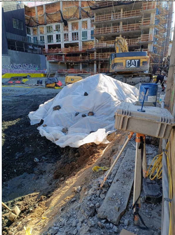
Photo 4- Representative photo of treated material stockpile pile covered with poly at the end of activities.
