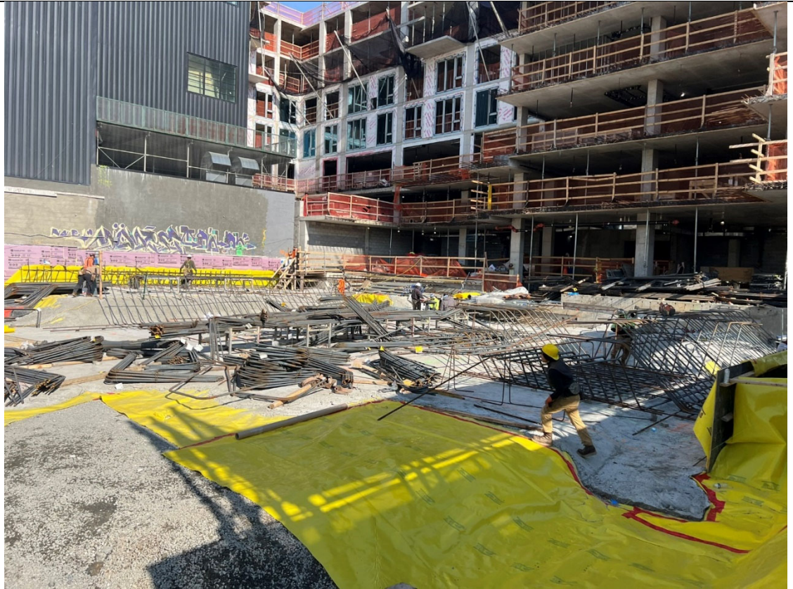
Photo 3- Representative photo of vapor rebar work.
