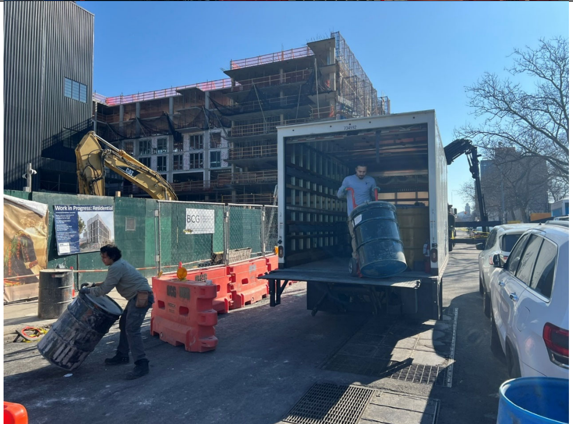
Photo 2- Representative photo of drums containing frac tank sediment being removed for offsite disposal.
