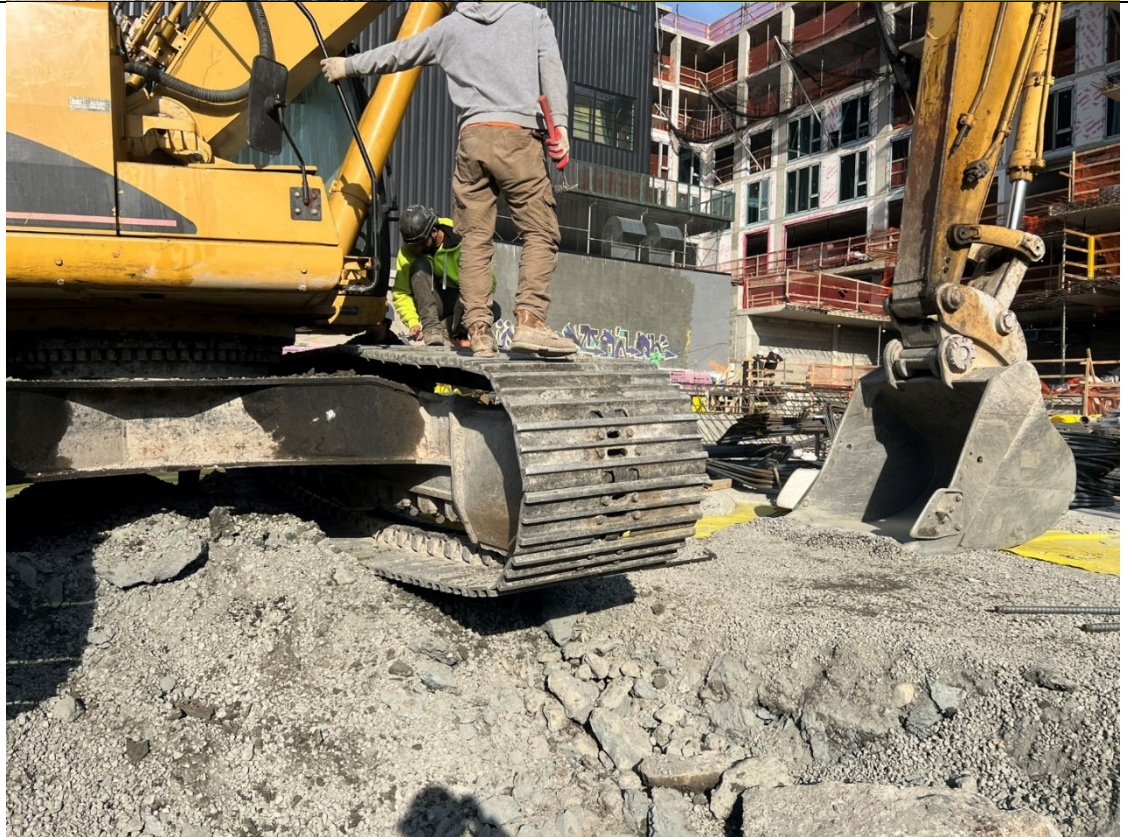
Photo 4- Representative photo of the cleaning excavator tracks.
