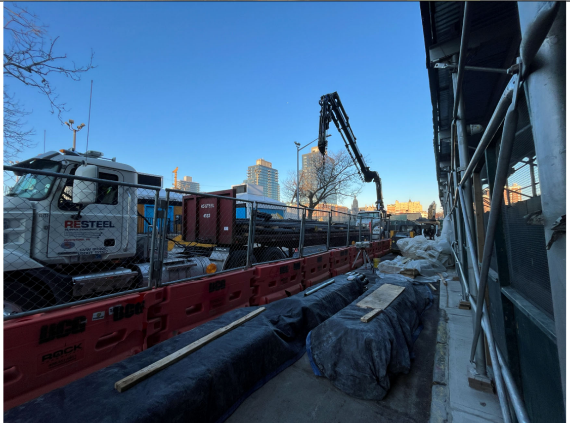
Photo 2- Representative photo of rebar truck on Douglass Street.
