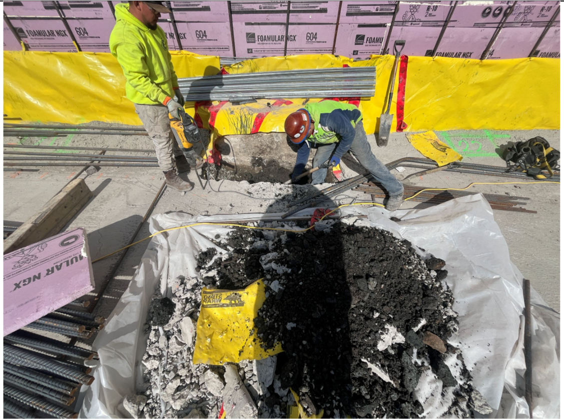
Photo 3- Representative photo of Concrete Courses digging around an adjacent property footing.
