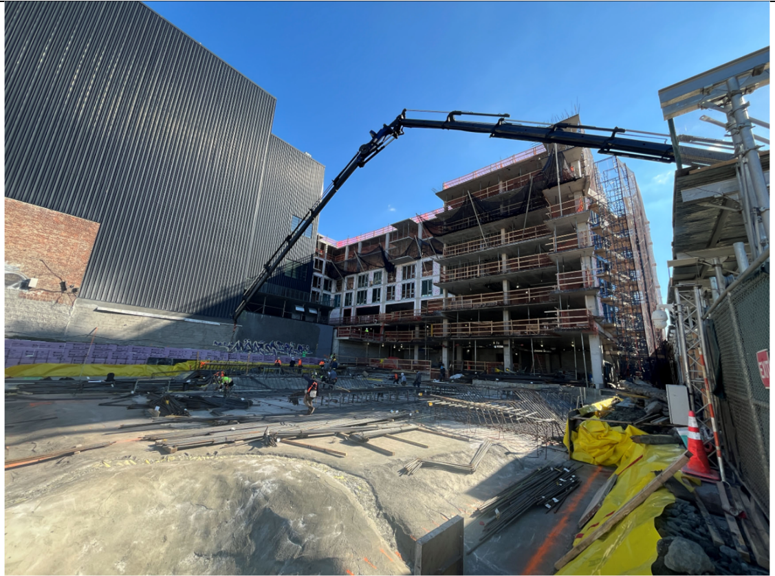
Photo 1- Representative photo of rebar delivery.
