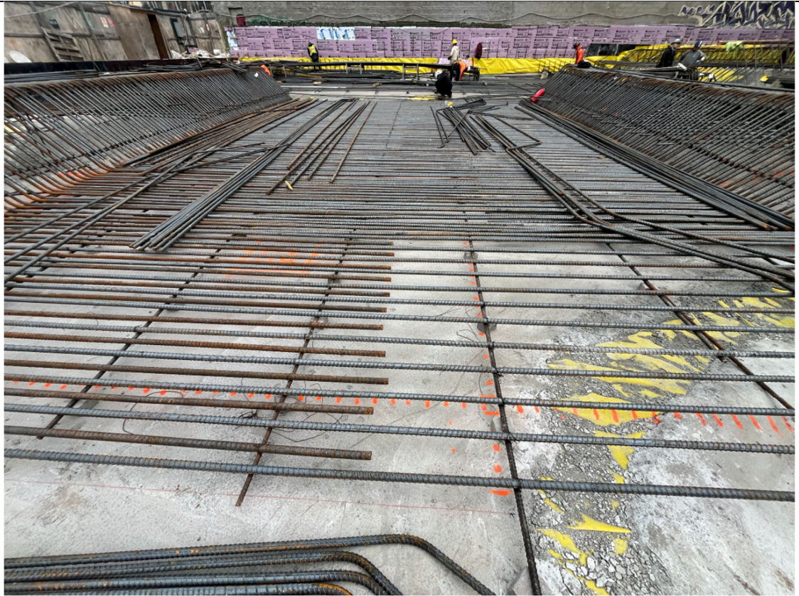
Photo 3- Representative photo of rebar installation.
