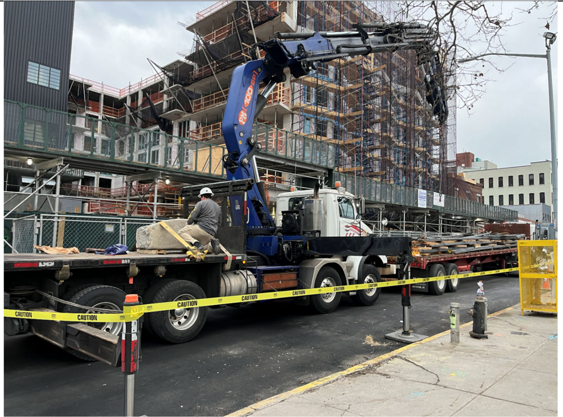
Photo 1- Representative photo of rebar delivery.
