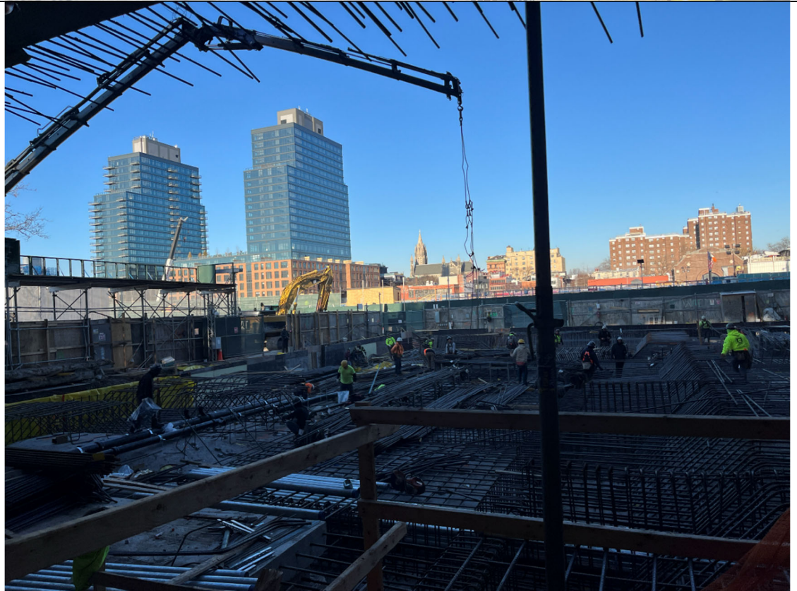
Photo 4- Representative photo of Concrete Courses moving rebar with crane.
