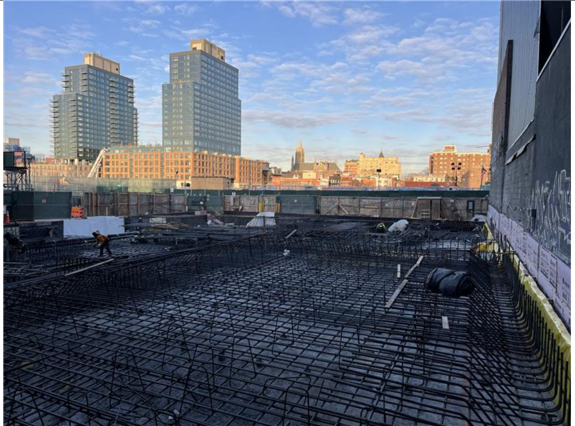
Photo 1- Representative view of the site facing west.
