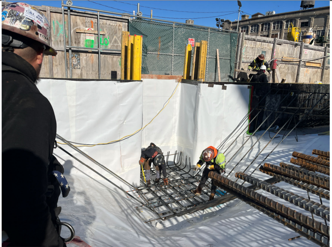
Photo 3- Representative photo of waterproofing adjacent to Nevins Street.
