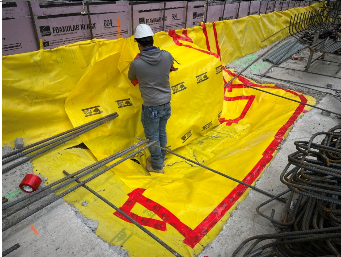
Photo 2- Representative photo of vapor barrier repair for footing in progress.
