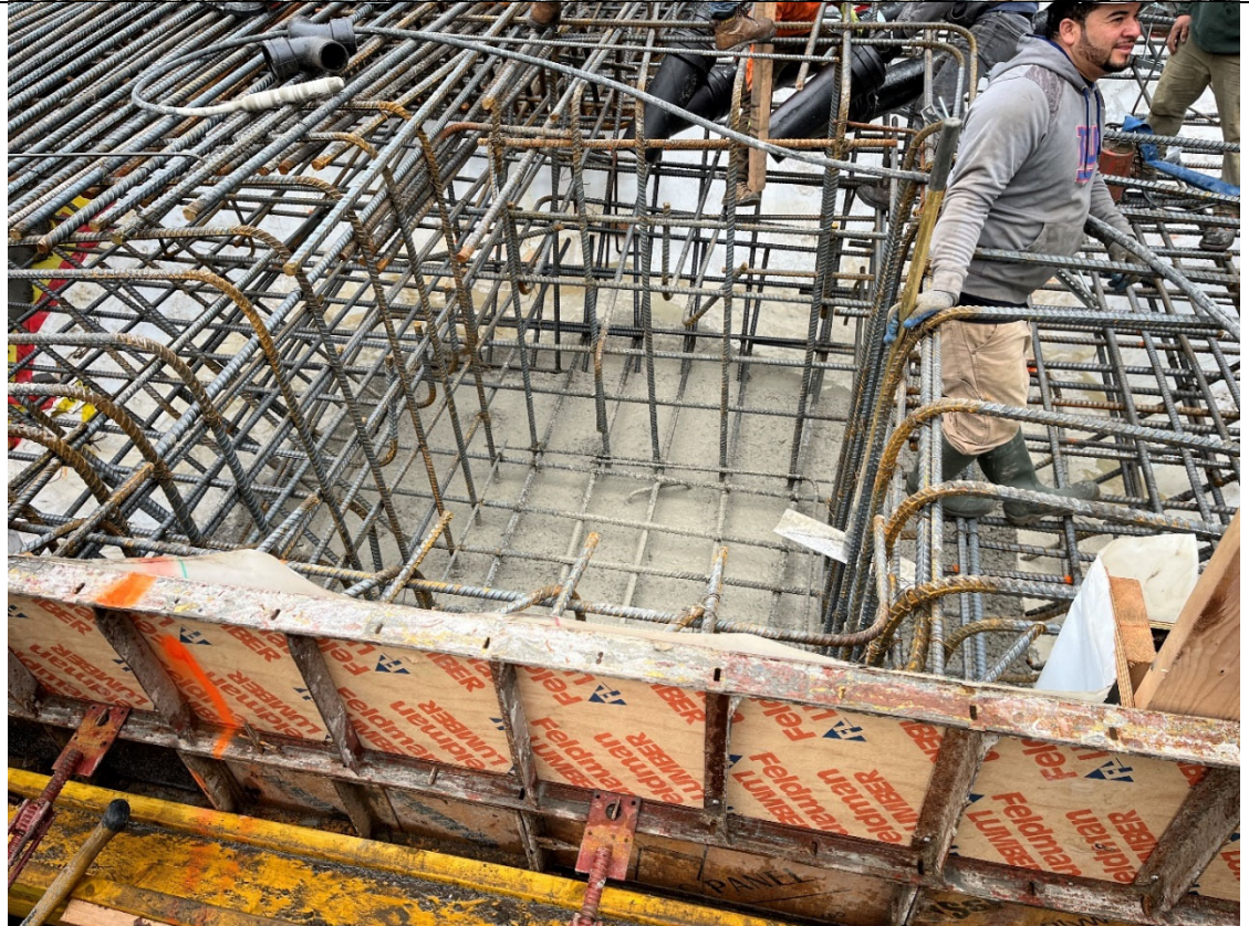
Photo 2- Representative photo of concrete pour.
