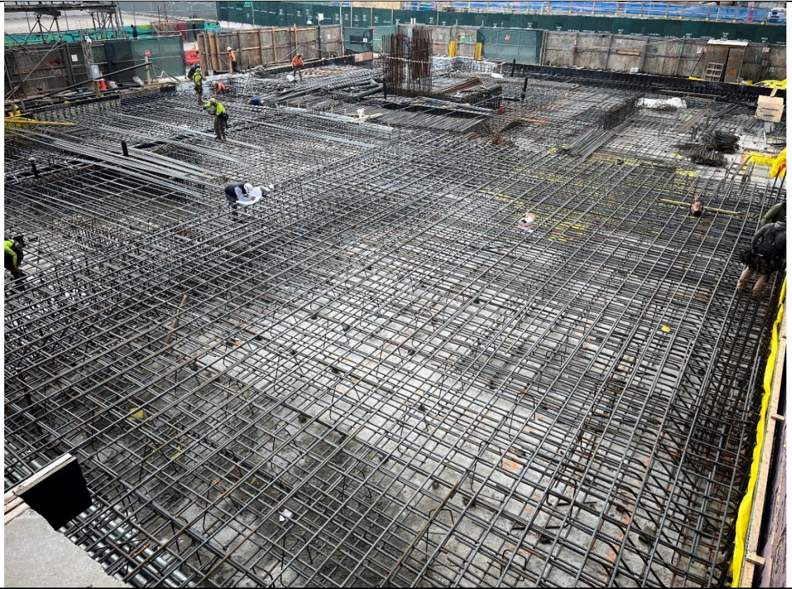
Photo 3- Representative photo of rebar work.
