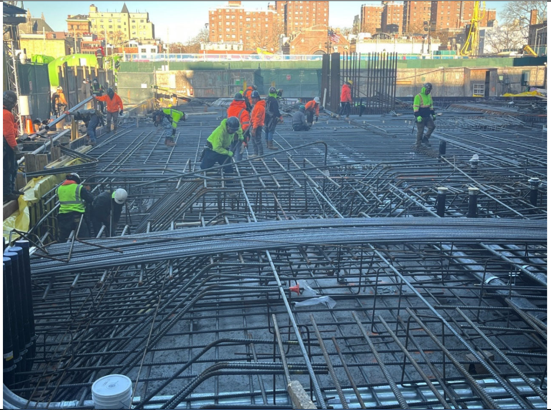
Photo 1- Representative view of the site facing west.
