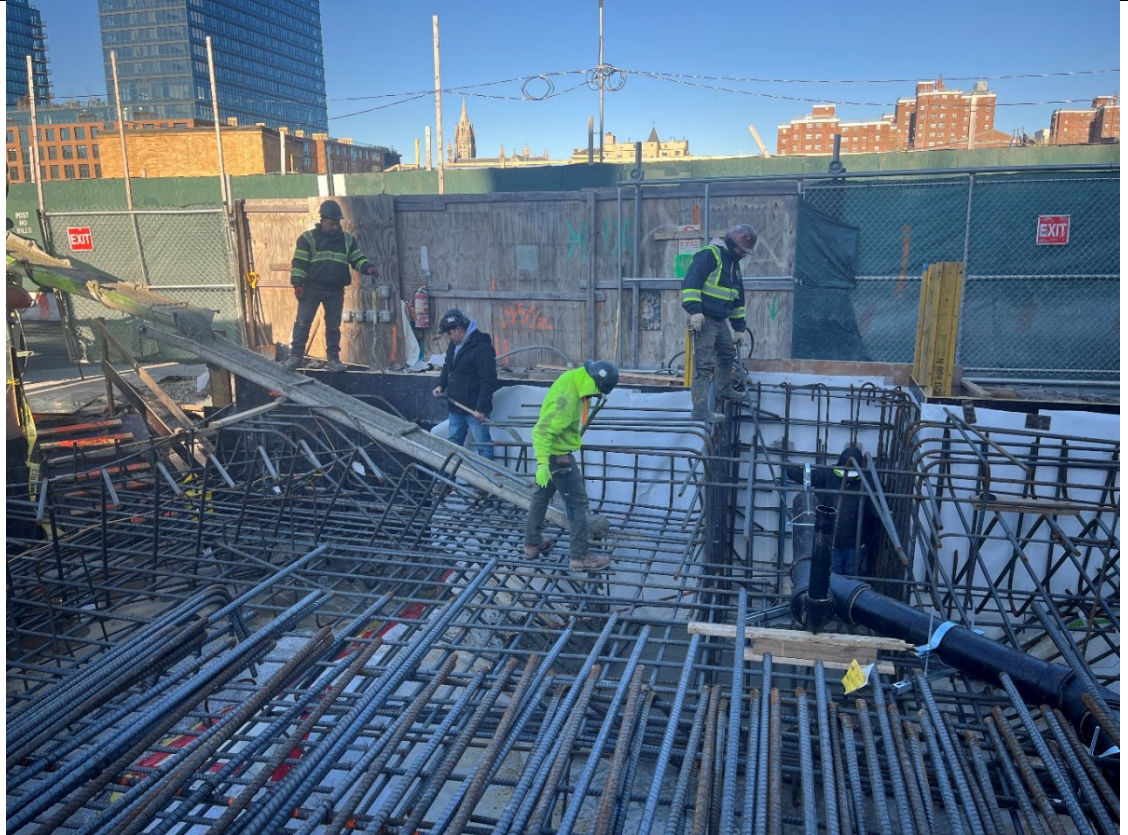
Photo 2- Representative photo of concrete pour.
