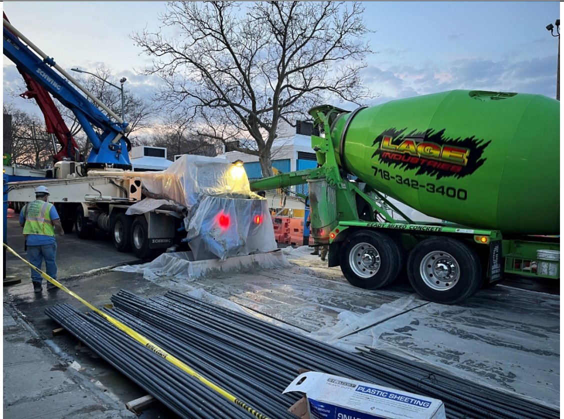
Photo 1- Representative view of the concrete pump setup.
