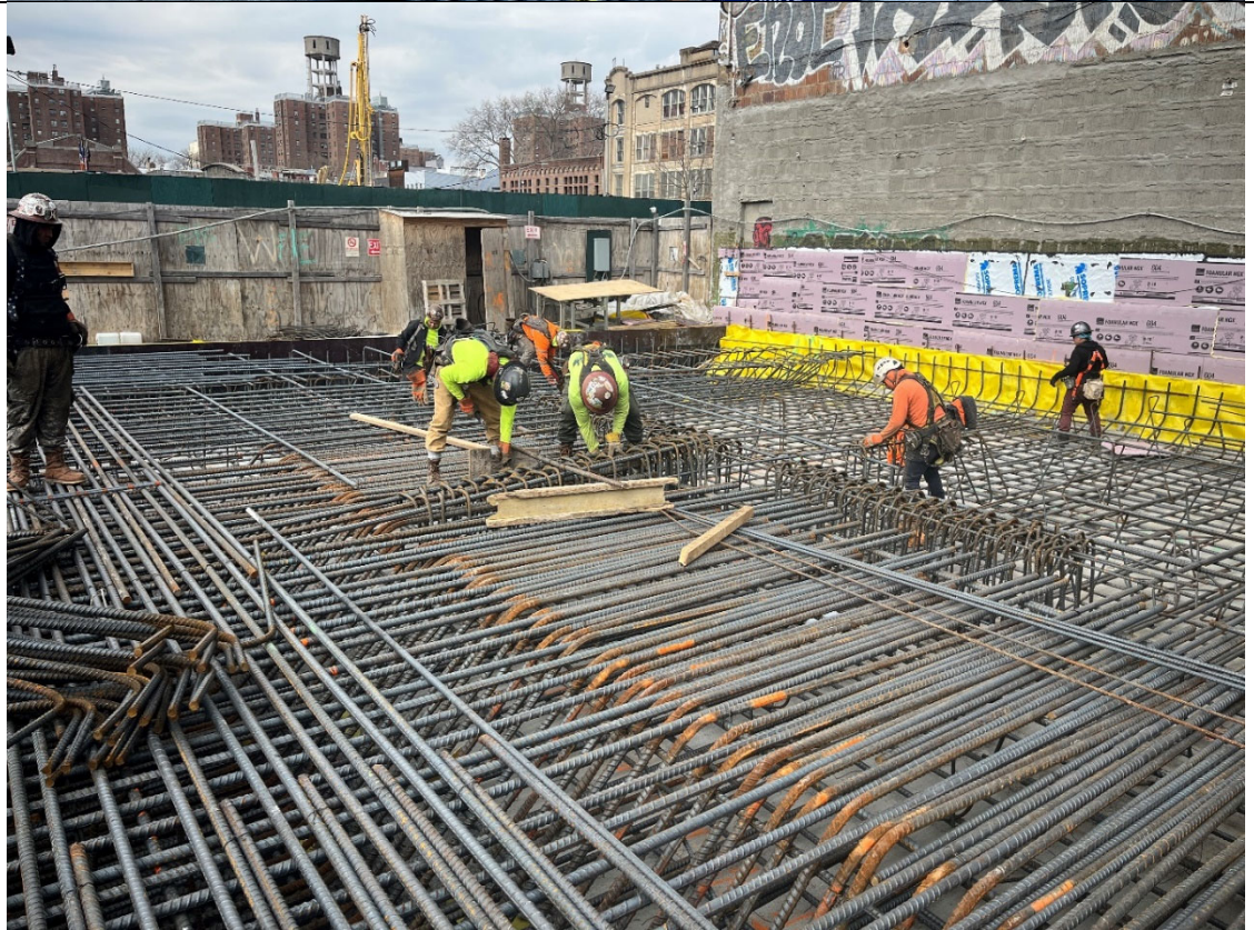
Photo 2- Representative photo of rebar work.
