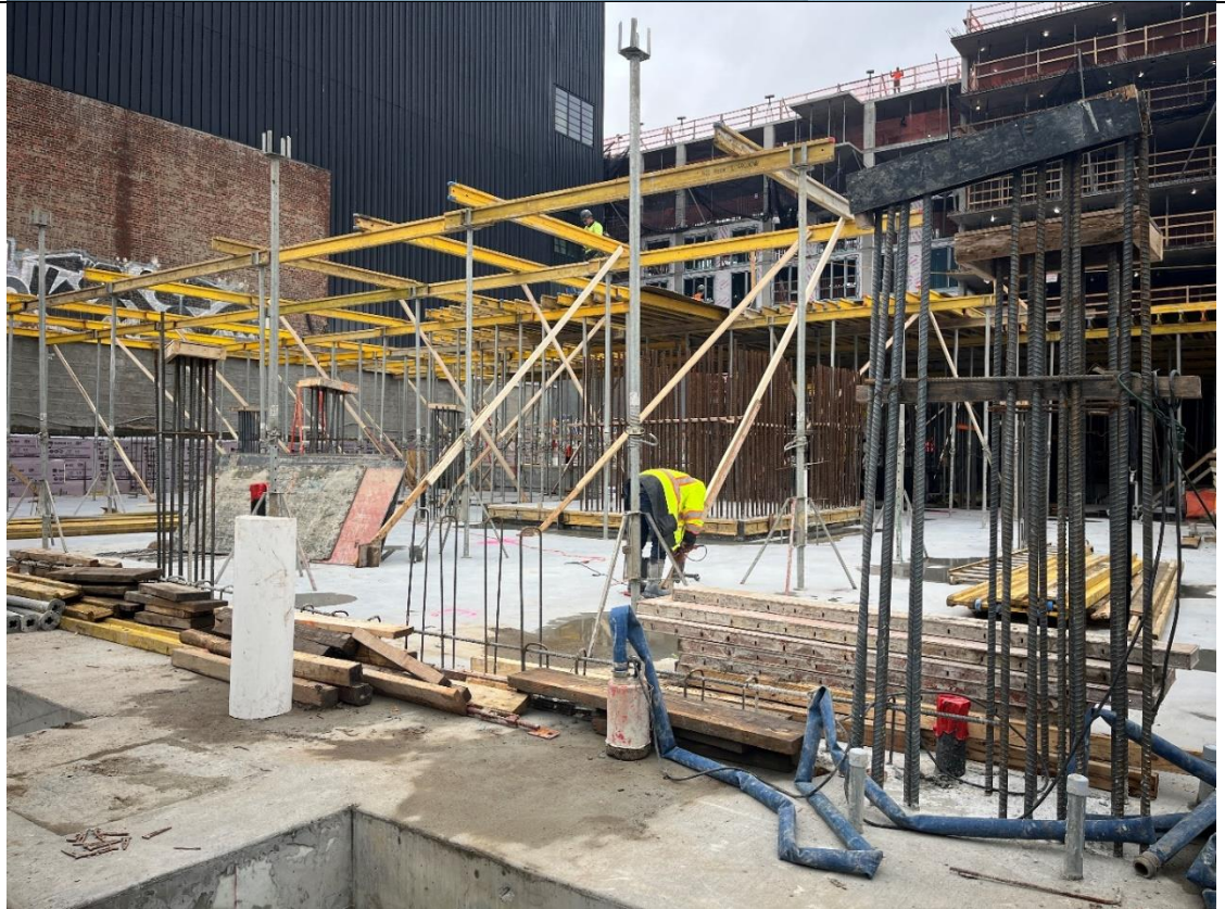
Photo 2- Representative photo of super structure work.
