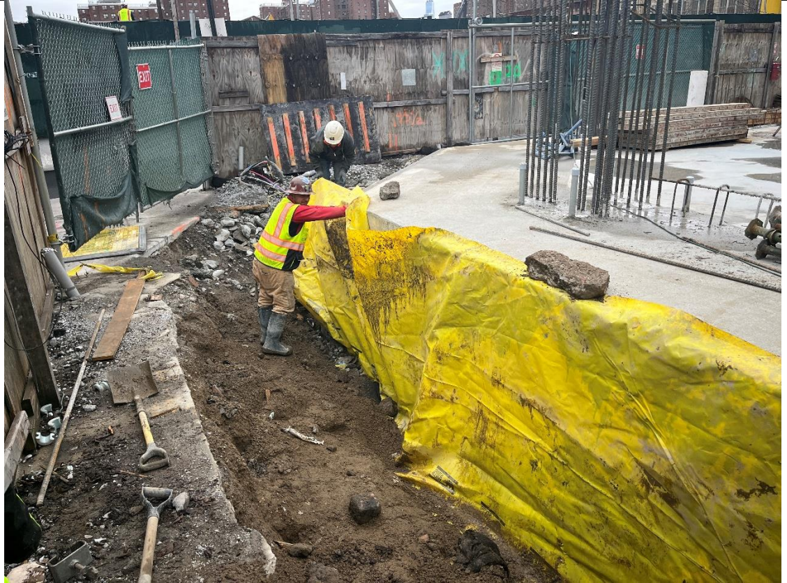
Photo 3- Representative view of the vapor barrier installation.
