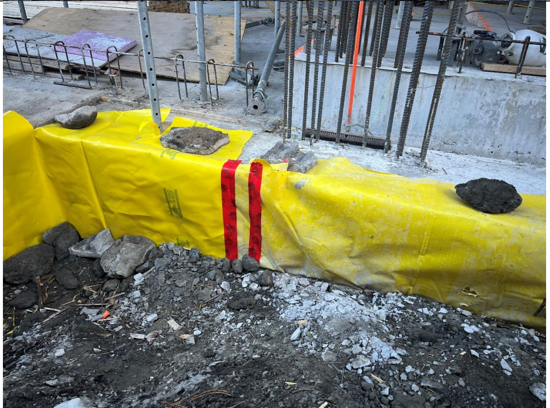
Photo 4- Representative view of the vapor barrier.
