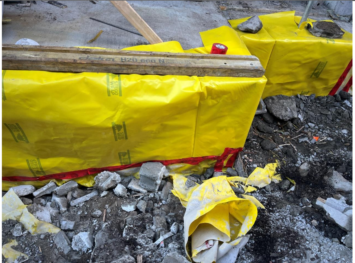
Photo 3- Representative view of the vapor barrier.
