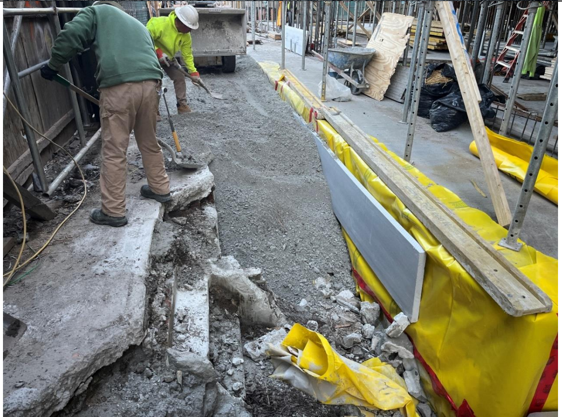
Photo 2- Representative photo of placing backfill around the mat-slab
