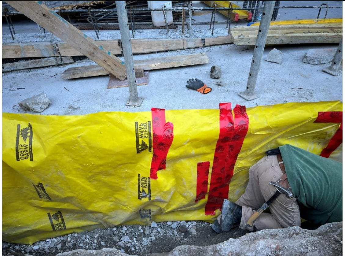
Photo 4- Representative view of the vapor barrier.
