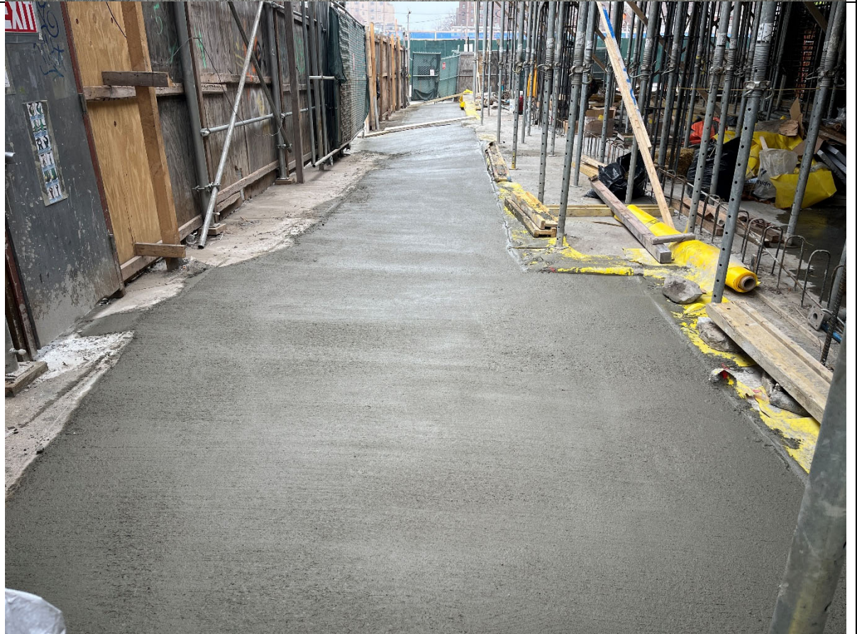
Photo 2- Representative photo of the concrete placement south of mat slab.
