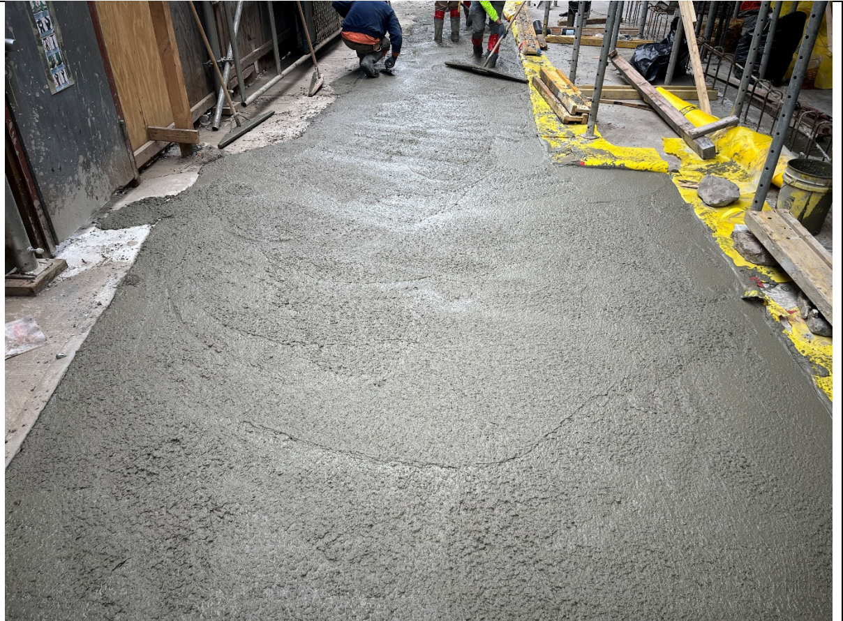
Photo 1- Representative view of the concrete placement.
