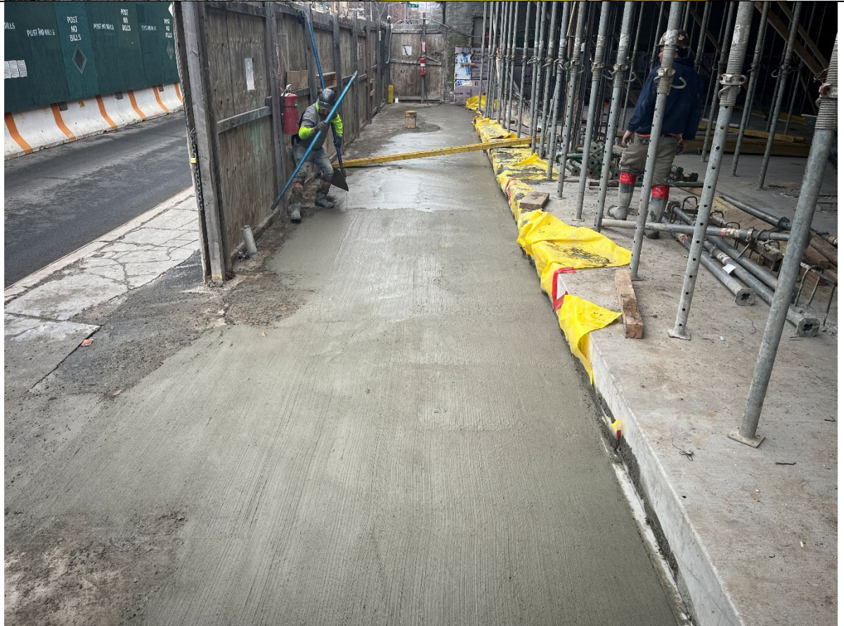
Photo 4- Representative view of finished concrete west of mat slab.
