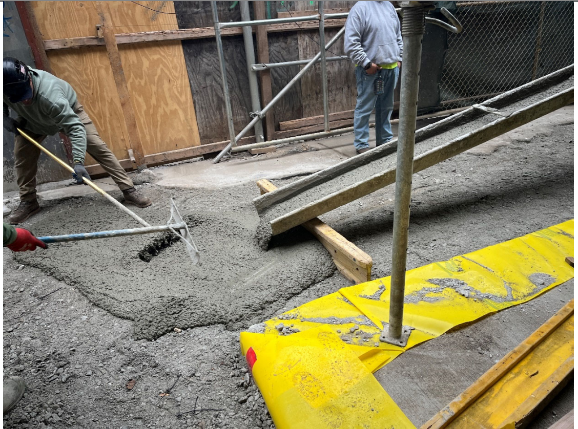
Photo 3- Representative view of the concrete placement.
