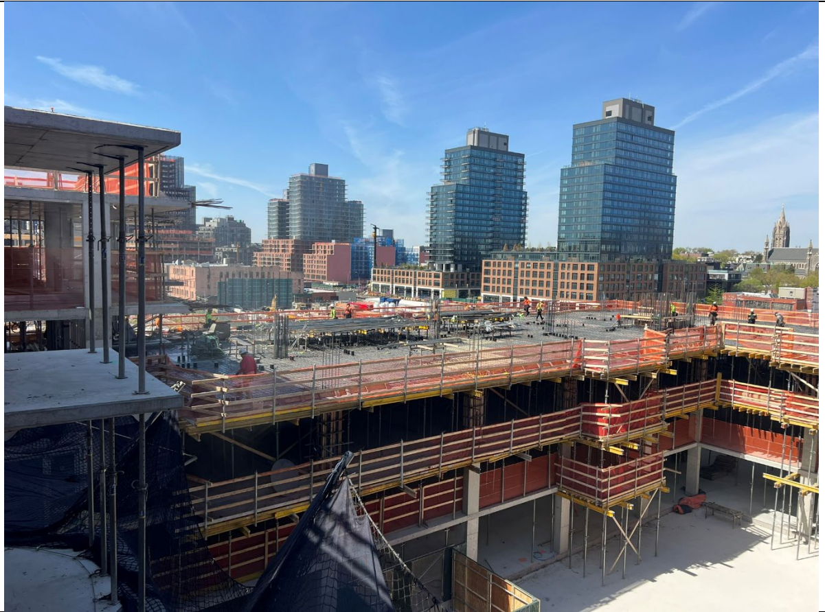
Photo 3- Representative view of 6 th floor being prepared for the concrete pour.
