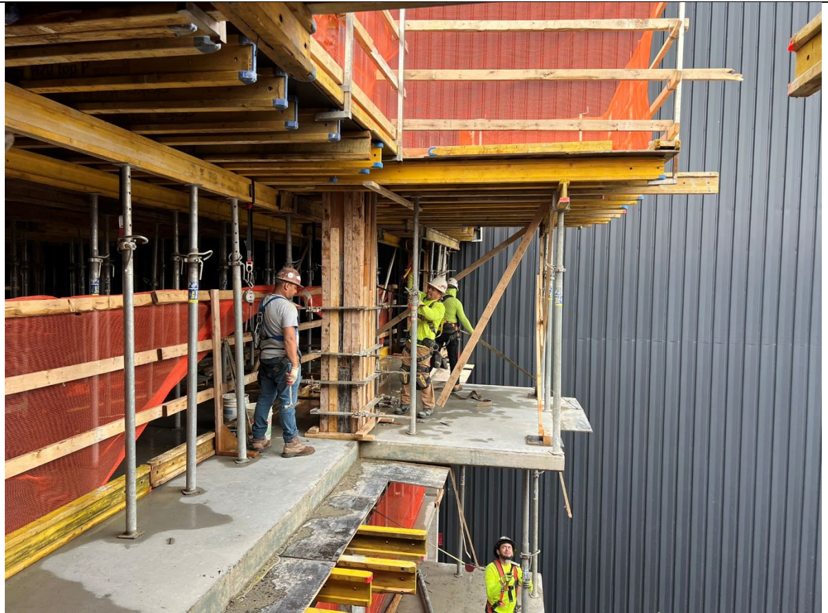
Photo 2- Representative photo of installing form work.
