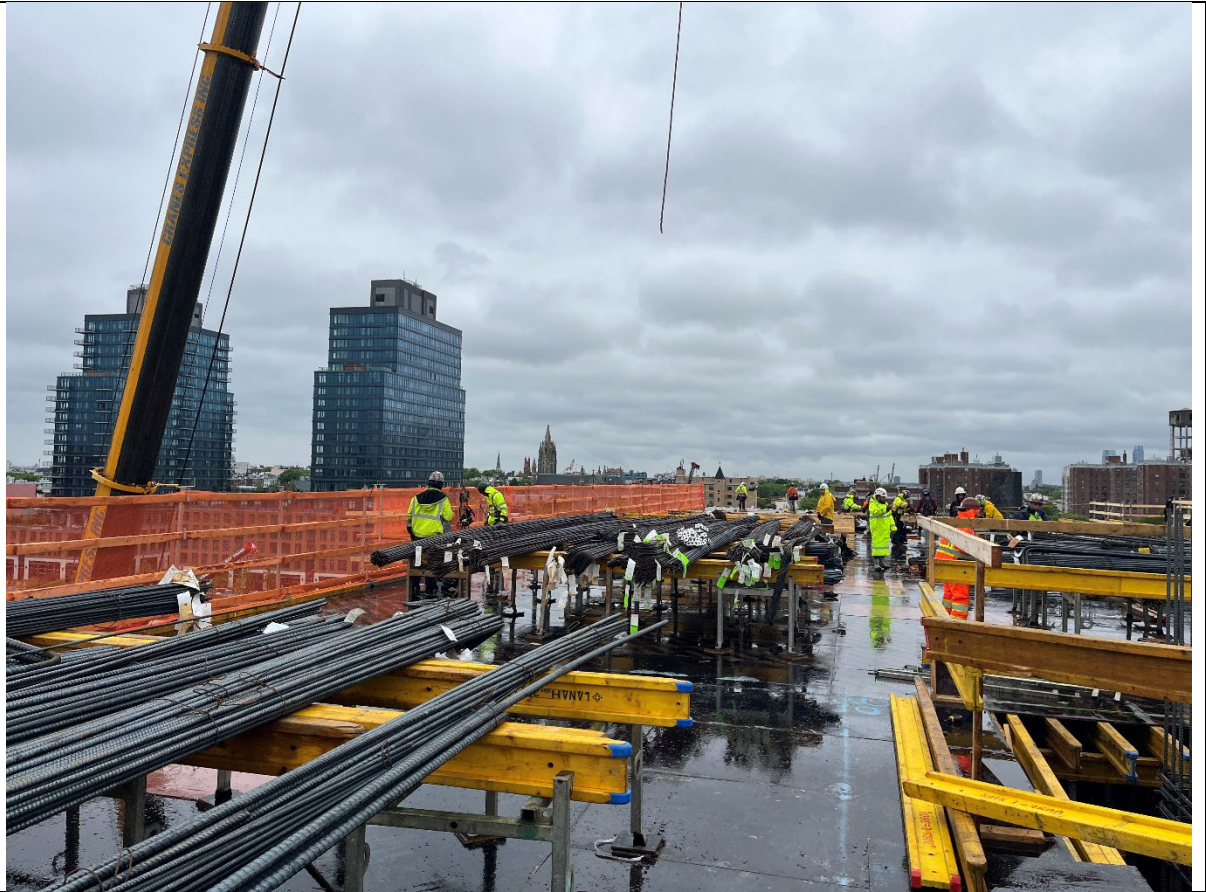
Photo 3- Representative view of form and rebar work for the 10 th story.
