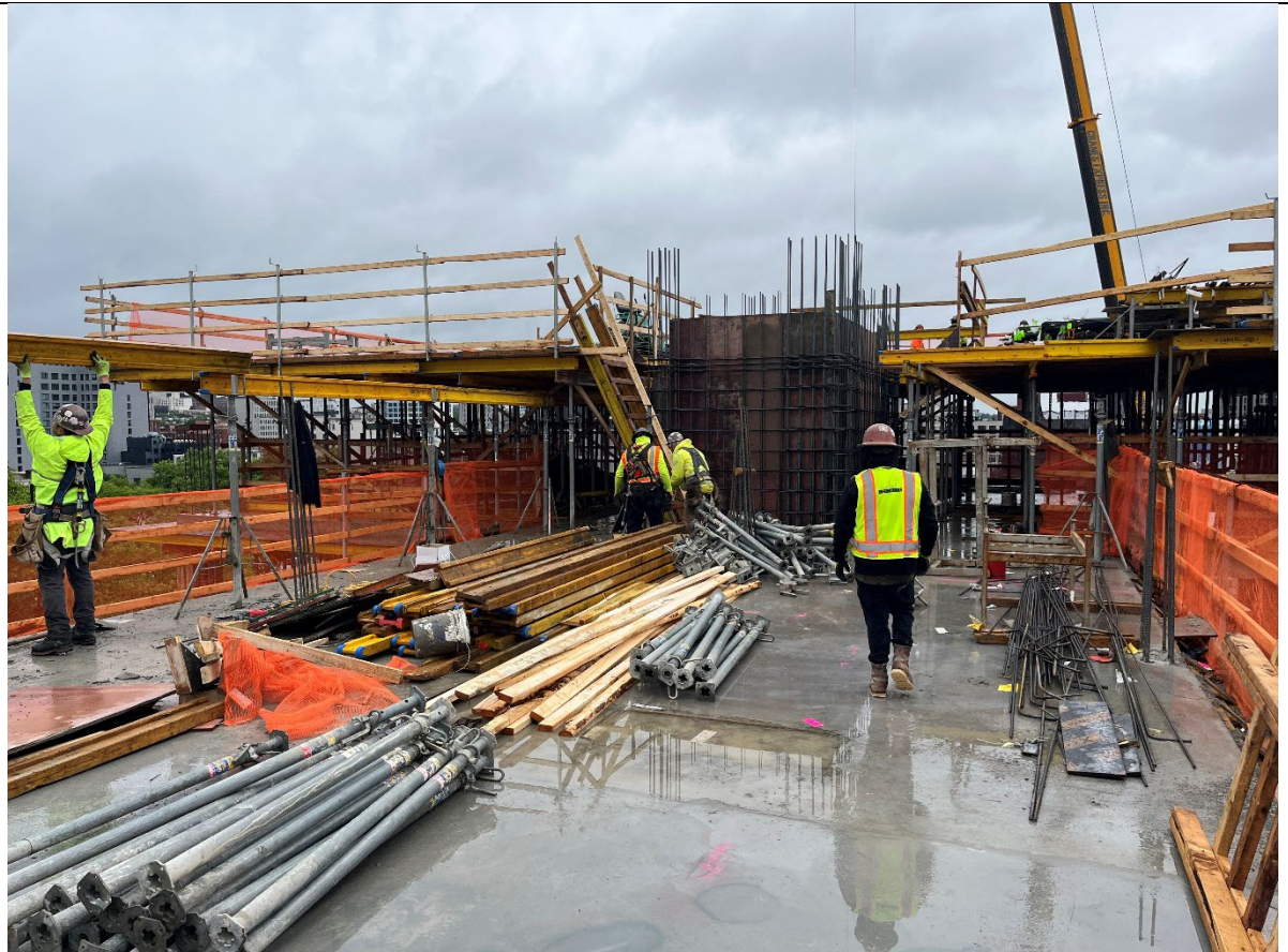
Photo 2- Representative photo of installing form work on 10 th story.
