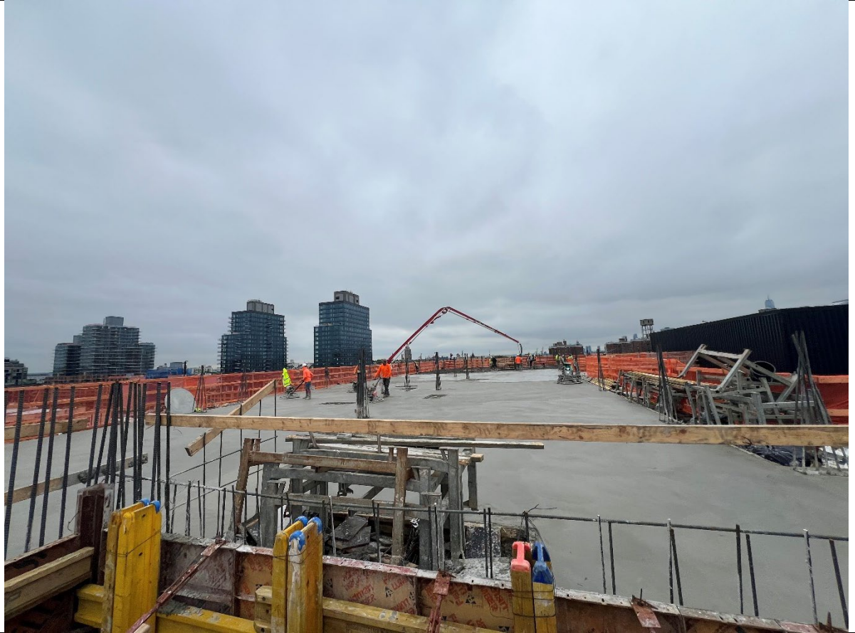
Photo 2- Representative photo of pouring concrete on 10 th story.
