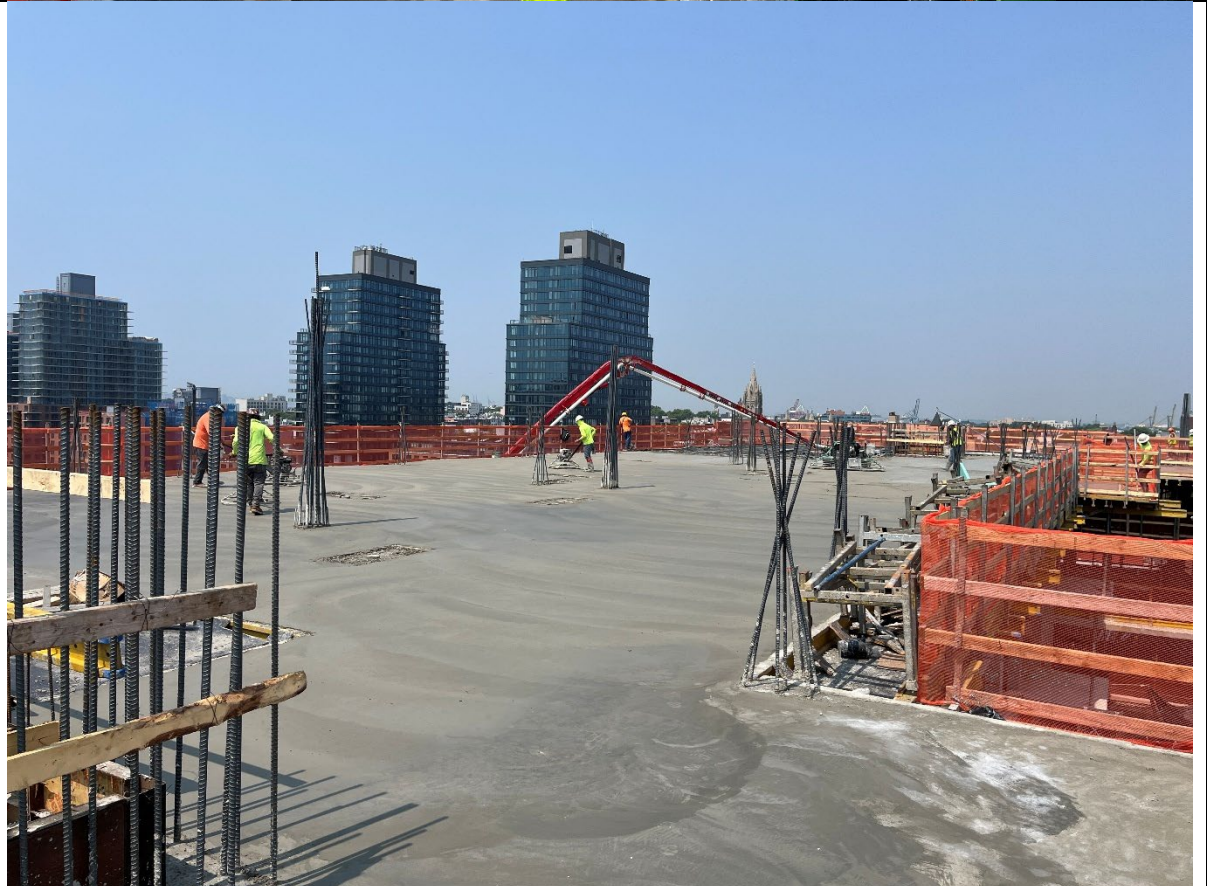
Photo 2- Representative photo of pouring concrete on 11 th story.
