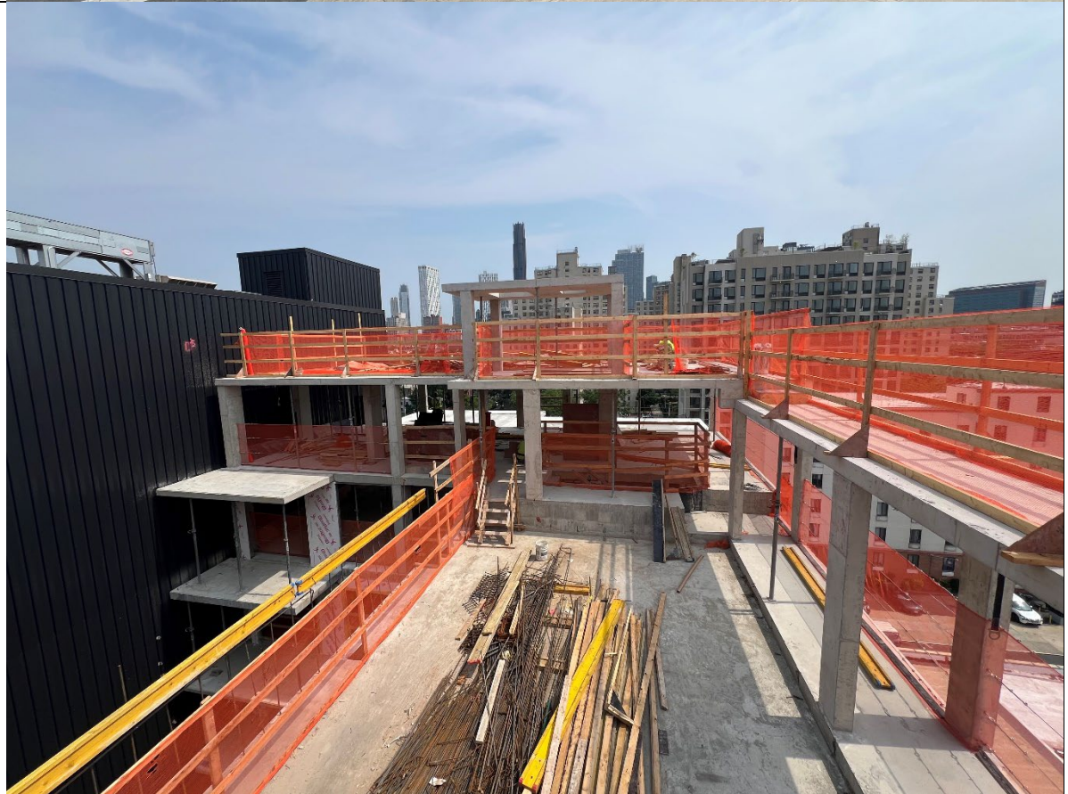
Photo 2- Representative photo of the completed 11 th story of the superstructure.
