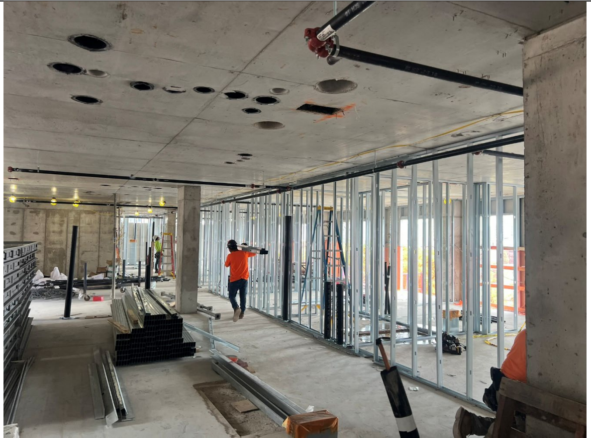
Photo 2- Representative photo of framing work.
