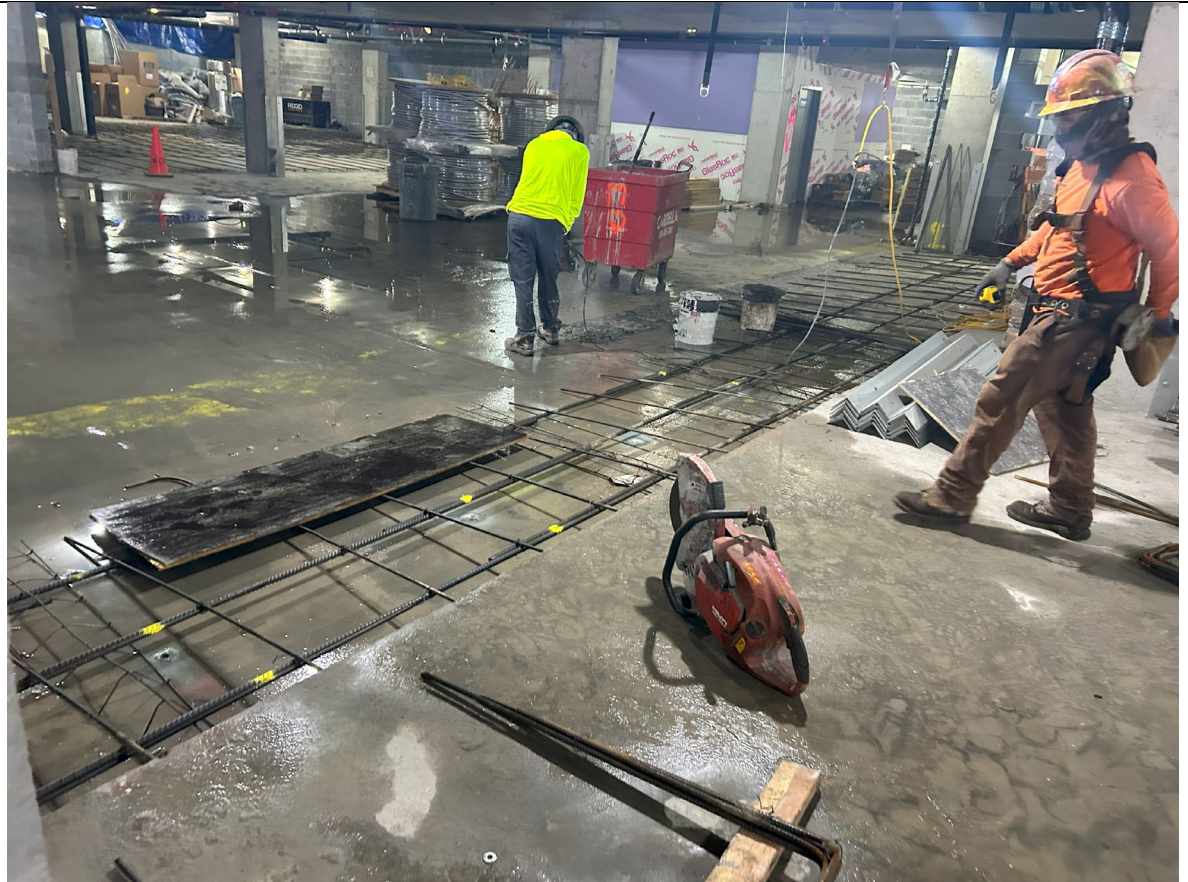
Photo 2- Representative photo of placing rebar for ramp construction on the second floor.
