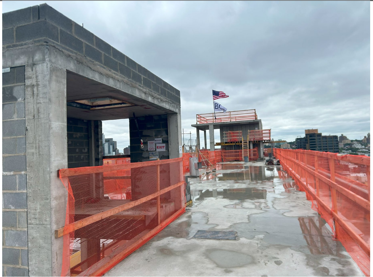
Photo 1- Representative view of the roof access.
