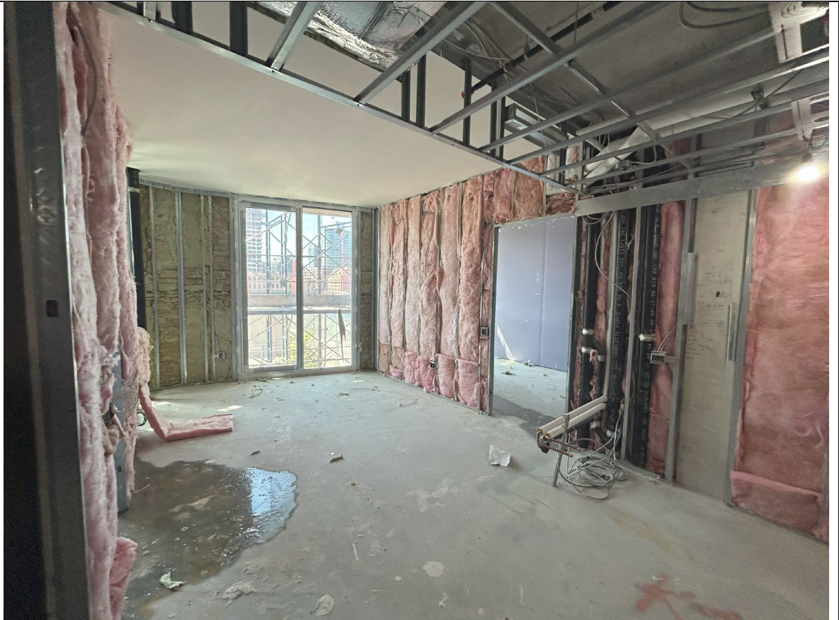
Photo 3- Representative view of insulation installed on the third floor.
