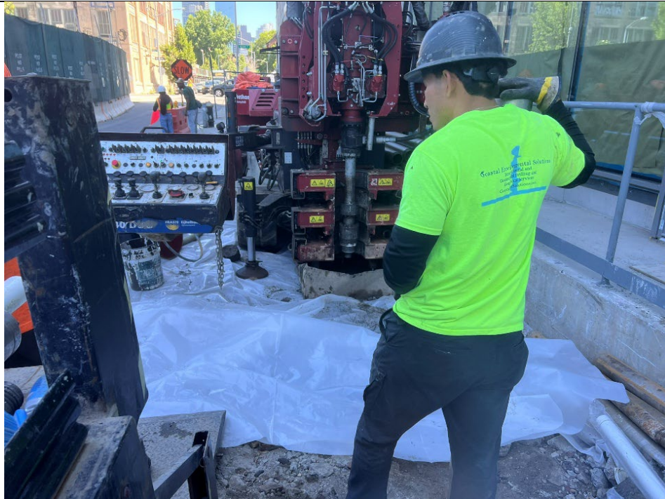
Photo 2 – Representative photo of drill rig set up at well OSMW-2B.
