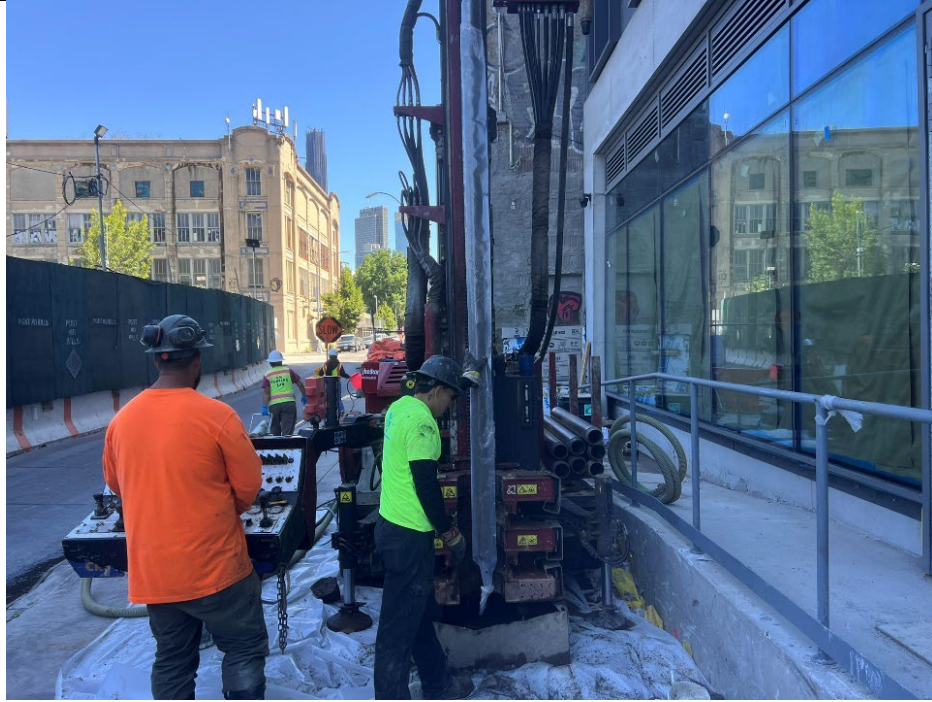
Photo 1- Representative photo of monitoring well installation activities at well, OSMW- 2A, located along Nevins Street.
