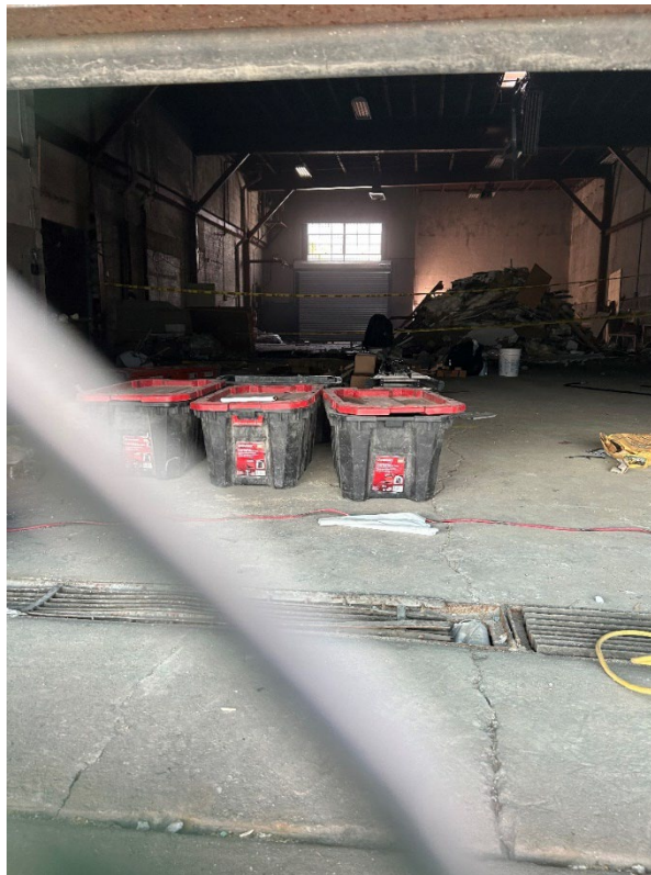
Photo 2: View of interior demolition.
