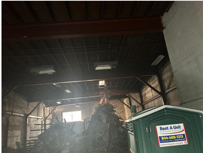
Photo 2: View of interior demolition, facing south.
