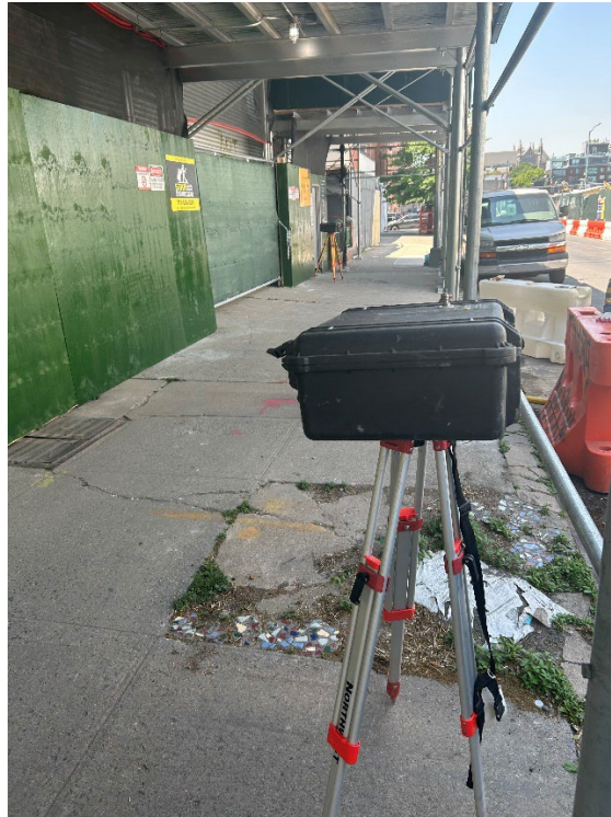
Photo 1: View of site exterior and CAMP setup, facing west.
