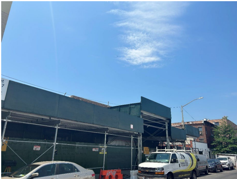
Photo 2: View of exterior demolition, facing south.
