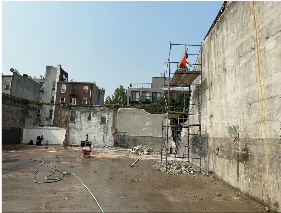
Photo 1: View of demolition activities, facing south.
