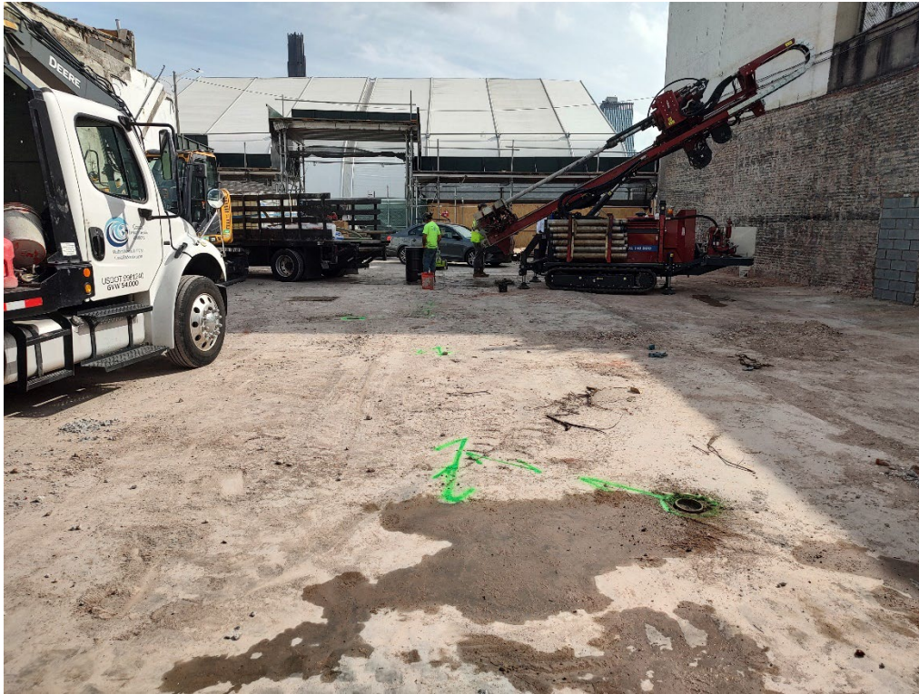
Photo 1 – Photo of the site during drilling operations showing the demolished lot. Multiple detections were located with GPR during the first investigation which were determined to be former storm drain utilities.
