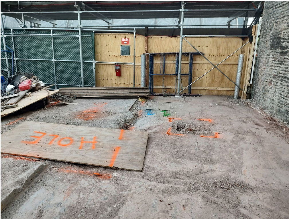
Photo 3 – Photo of the partially backfilled basements present on site which were covered and labeled for safety. Also visible in this photo are the disconnected lines formerly used for water (blue) and sewer (green) utilities.
