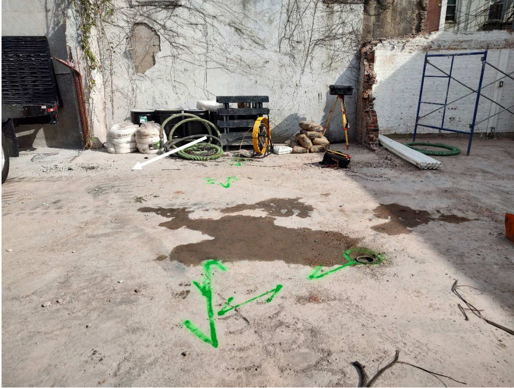
Photo 2 – Additional drainage structures identified in the field.
