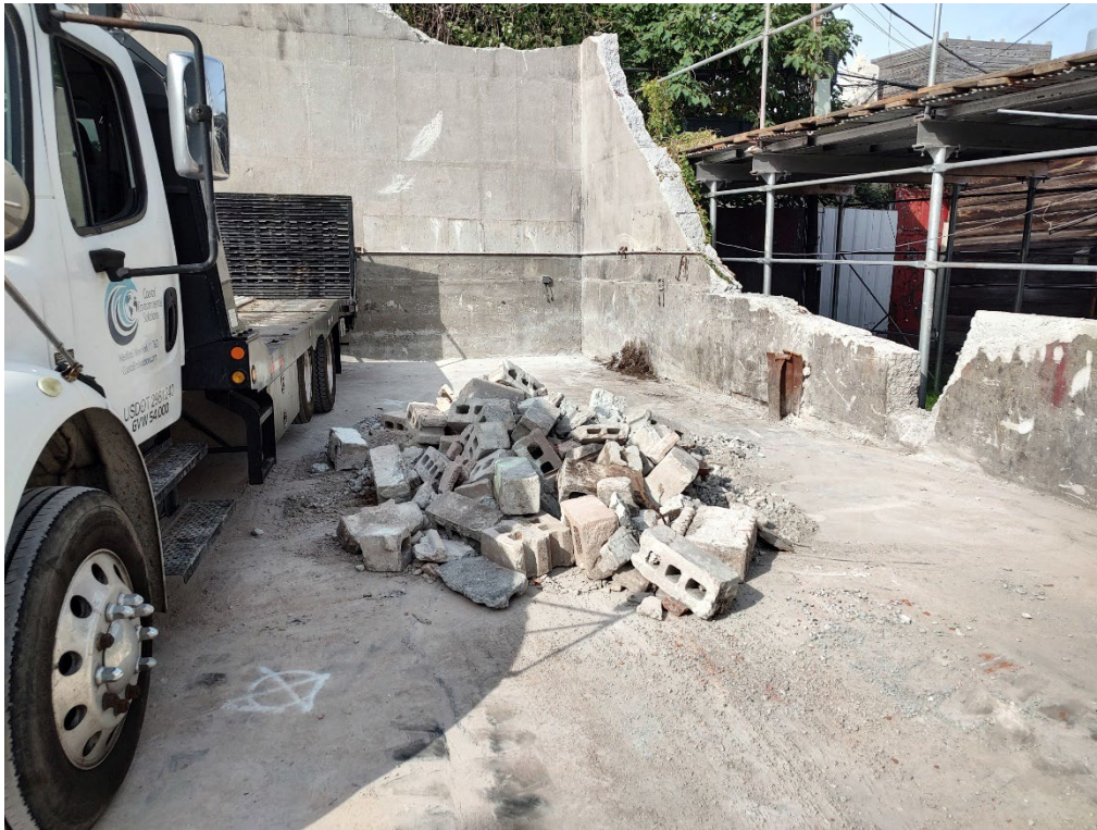
Photo 4 – Photo of one of the debris piles present which prevented subsurface investigation in their immediate area. GPR scans were performed by Coastal around this debris pile to determine the absence of any utilities.
