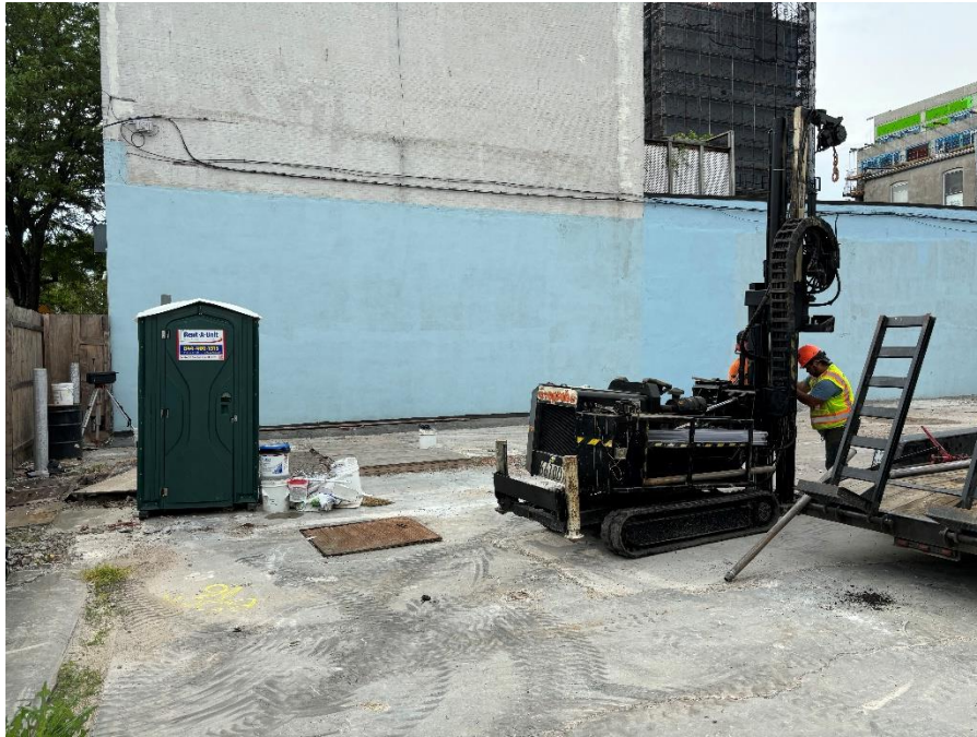
Photo 1: Contractor drilling waste characterization boring, facing West.
