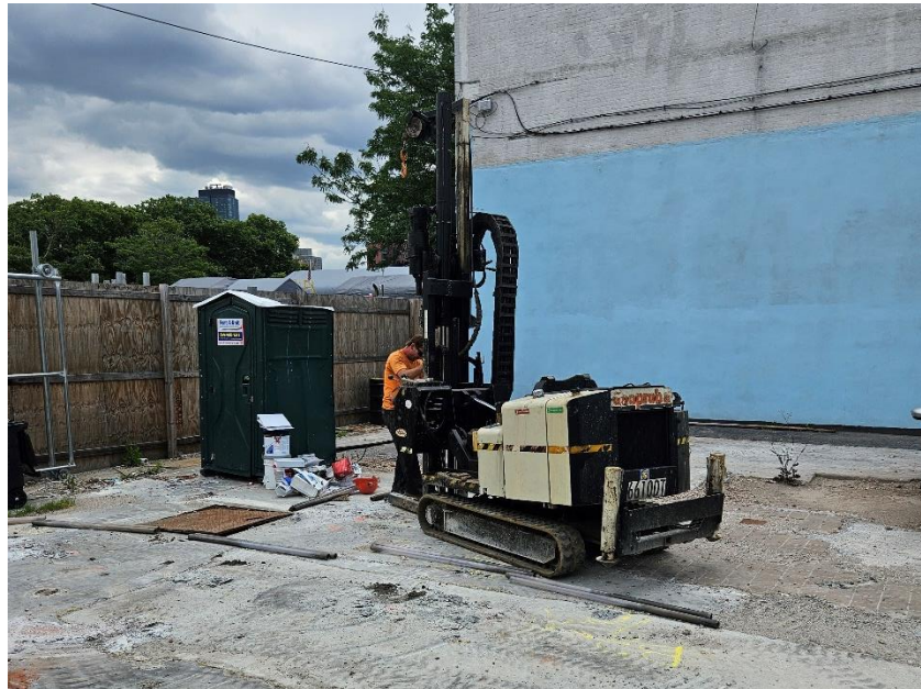
Photo 2: Contractor drilling lead delineation soil boring, facing Northeast.
