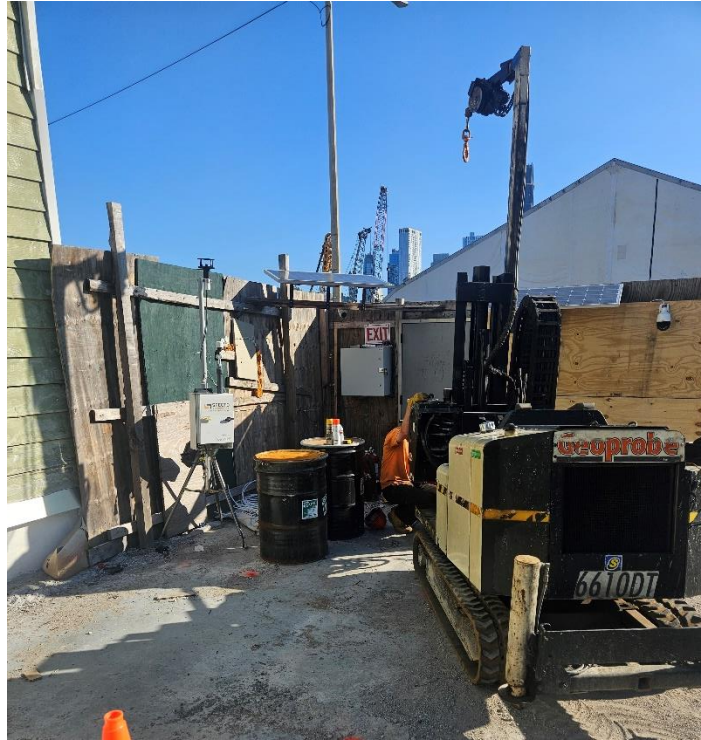
Photo 1: Contractor drilling lead delineation soil boring, facing Northwest.
