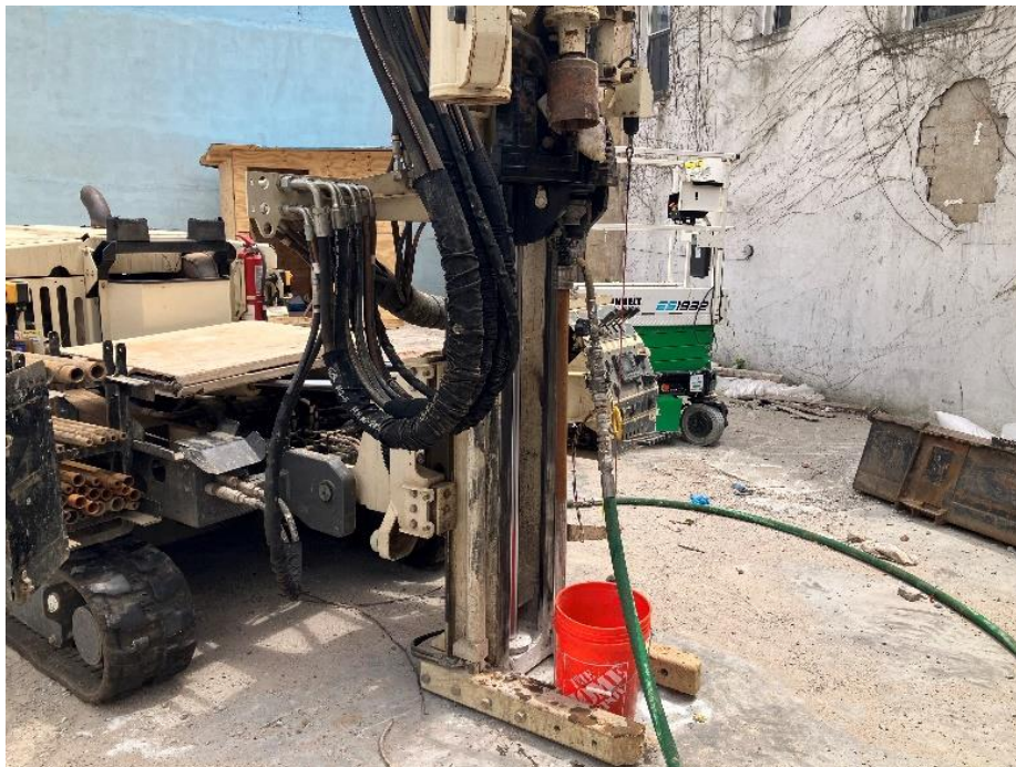
Photo 2: View of AWT installing ISCO injections in the southern portion of the Site, facing Southeast.
