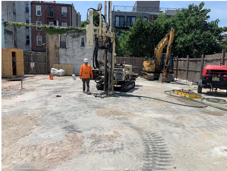
Photo 1: View of contractor drilling injection points/injecting persulfate, facing south.
