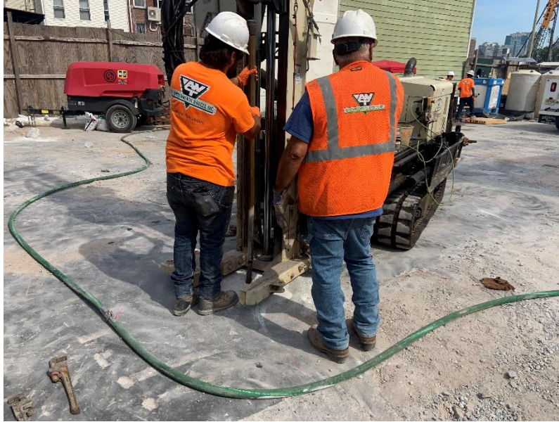
Photo 1: View of contractor drilling injection points, facing northwest.
