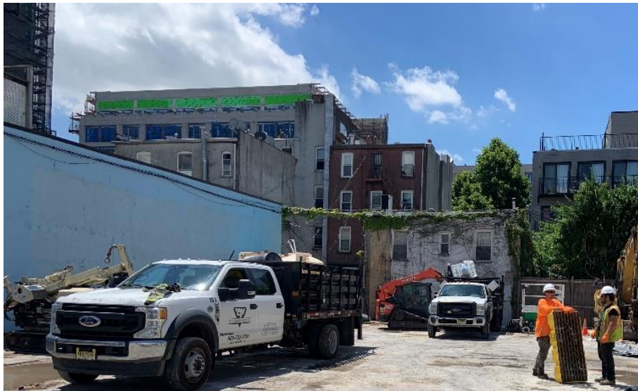
Photo 2: View of contractor demobilizing from the Site, facing south.
