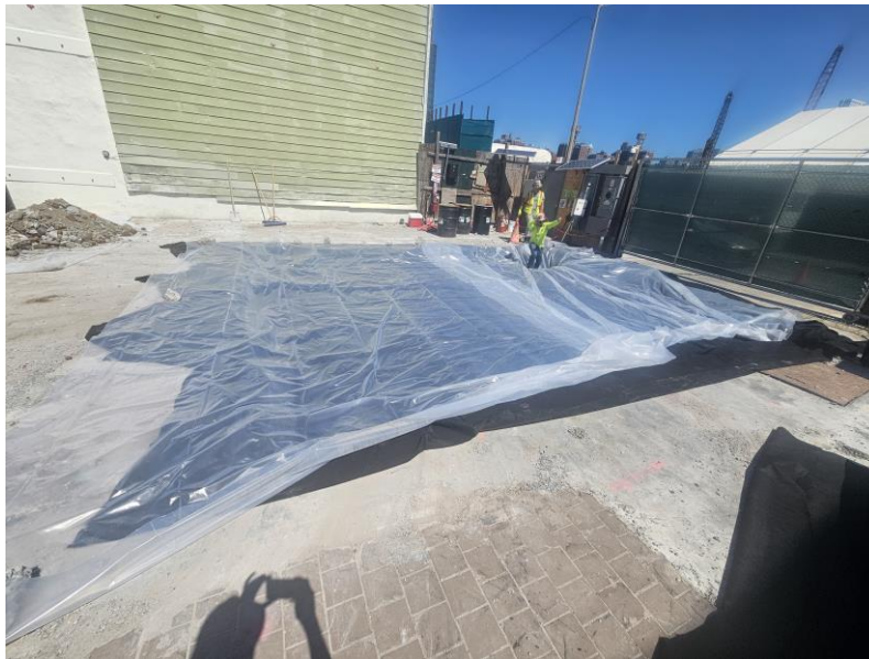
Photo 2: View of truck pad installation with polyethylene sheeting and geotextile fabric, facing west.
