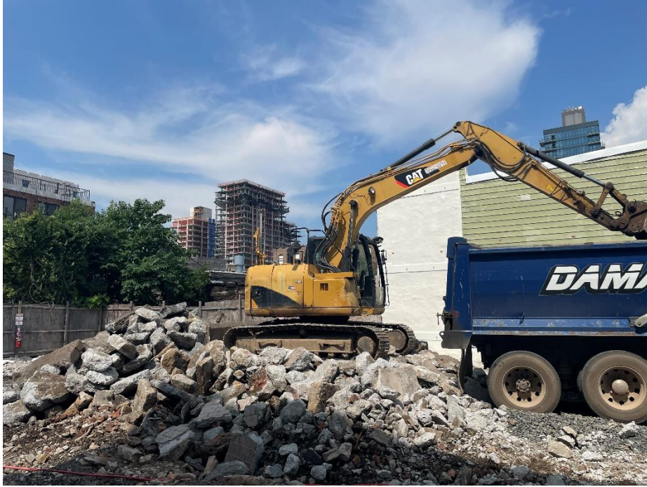
Photo 1: View of contractor loading C&D debris for disposal, facing southwest.
