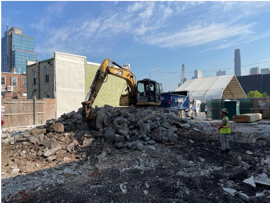
Photo 2: View of contractors stockpiling concrete for disposal, facing north.
