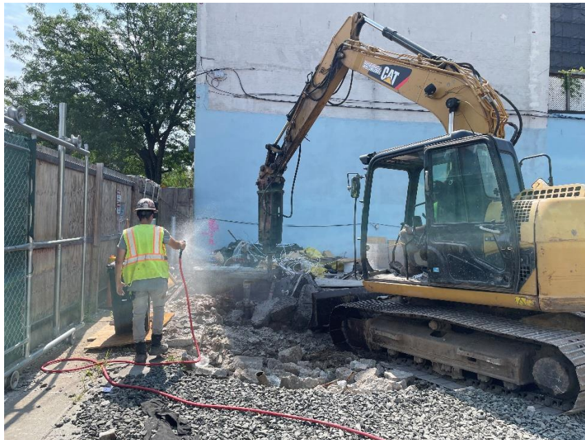
Photo 2: Water spray during concrete slab removal
