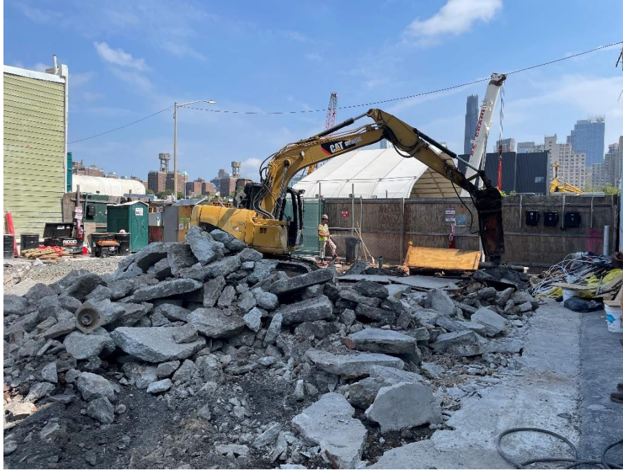
Photo 1: View of contractor breaking up concrete slab for disposal, facing north.
