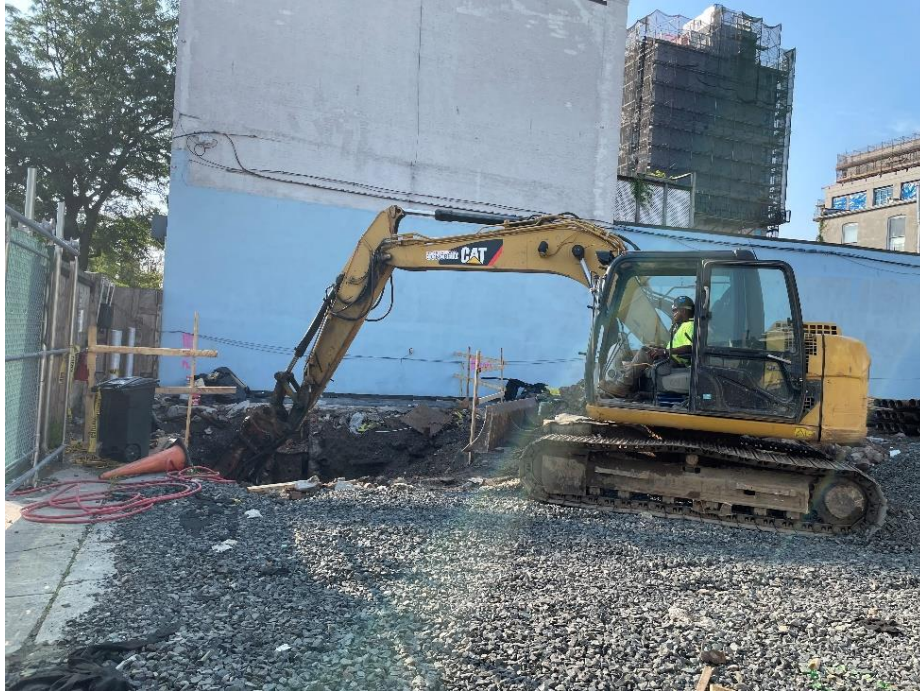
Photo 1: View of contractor breaking up concrete for disposal, facing east.
