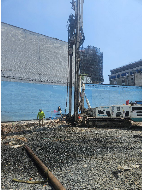
Photo 1: View of contractor installing piles for SOE, facing northeast.
