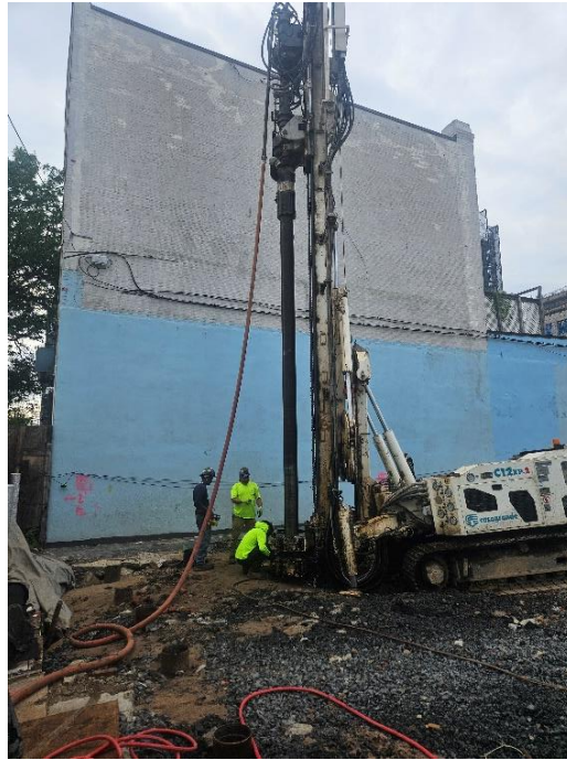
Photo 1: View of contractor installing piles for SOE, facing east.
