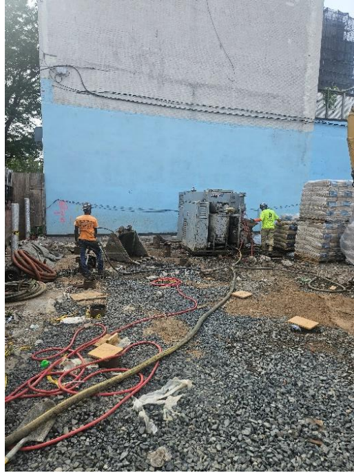
Photo 1: View of pile grouting, facing east.
