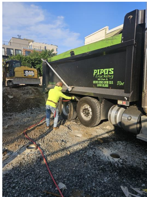
Photo 2: View of laborer cleaning truck undercarriage prior to departure, facing Southwest.
