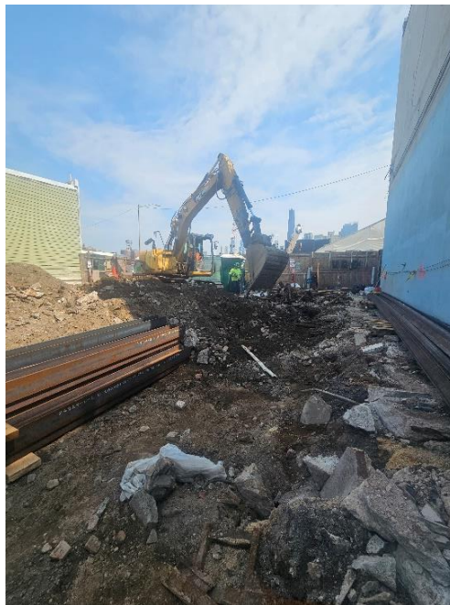
Photo 2: View of contractor stockpiling soil for off-Site disposal, facing Northwest.
