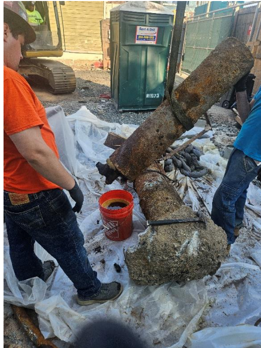
Photo 1: View of contractor draining hydraulic lift found on site, facing West.
