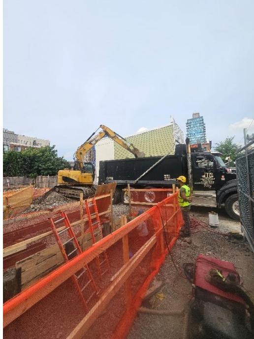
Photo 1: View of contractor loading soil for off-Site disposal, facing West.
