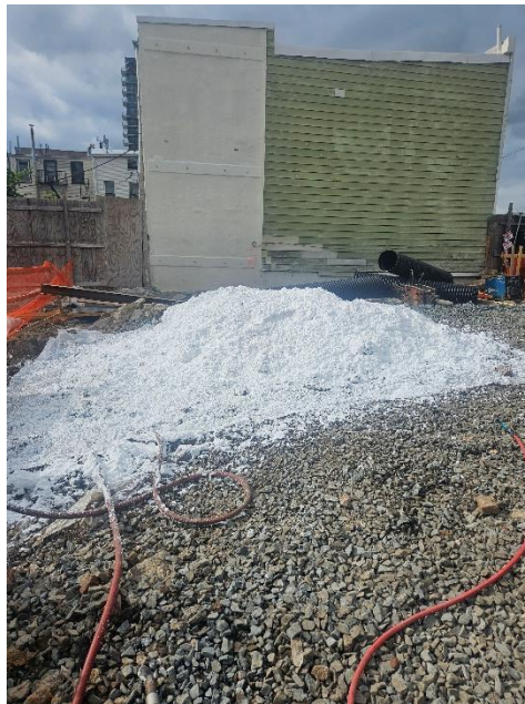
Photo 2: View of soil stockpile covered with odor control foam, facing West.
