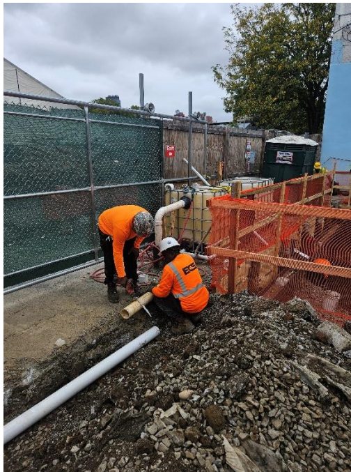
Photo 2: View of contractor installing dewatering system, facing Northeast.
